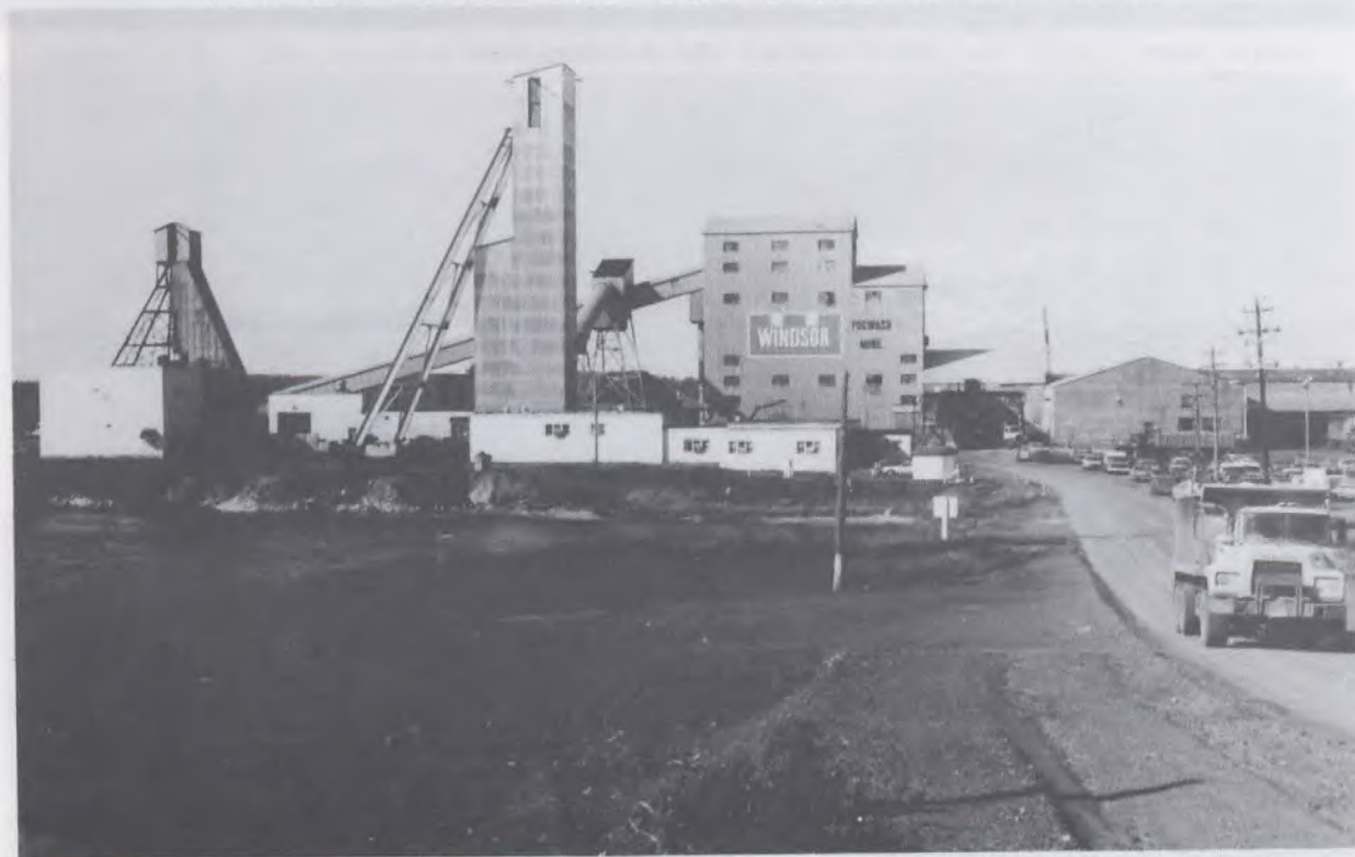
Canadian Salt Company Limited, Pugwash Mine, No. 1 head frame (left), No. 2 head frame (centre), Pugwash, Nova Scotia (October, 1980).
