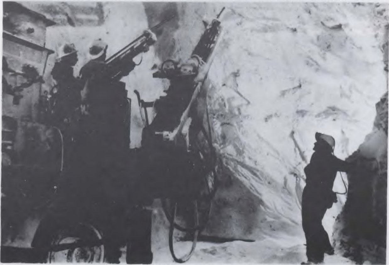
Drill used to drill blast holes in mining face, Pugwash Mine (NSIS).
