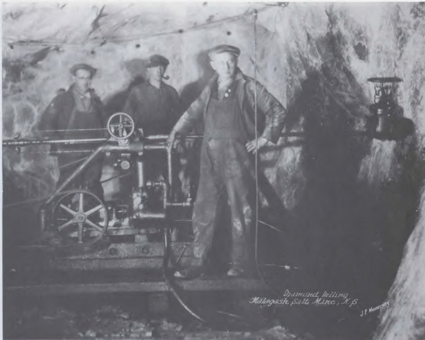
Diamond-drilling at face of Lucas Seam, No. 3 West Level, 500 feet from main slope, Malagash Mine, November 20, 1929.
