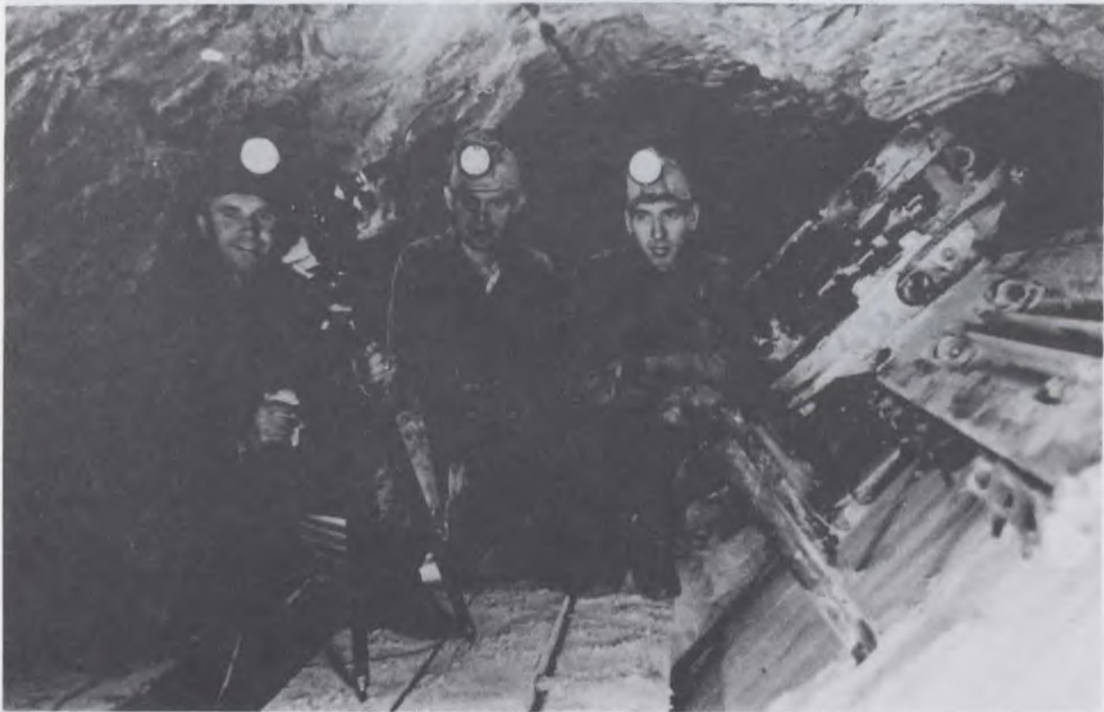
Undercutting a mine face (stope and level unknown) Malagash Mine (courtesy Reid Picture and Equipment Service).
