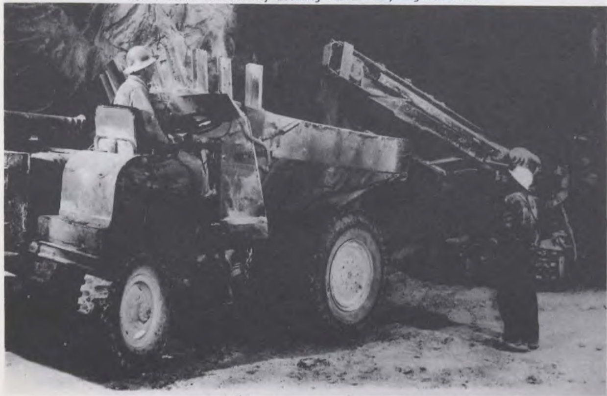
Loading salt into haulage trucks, Pugwash Mine (NSIS).
