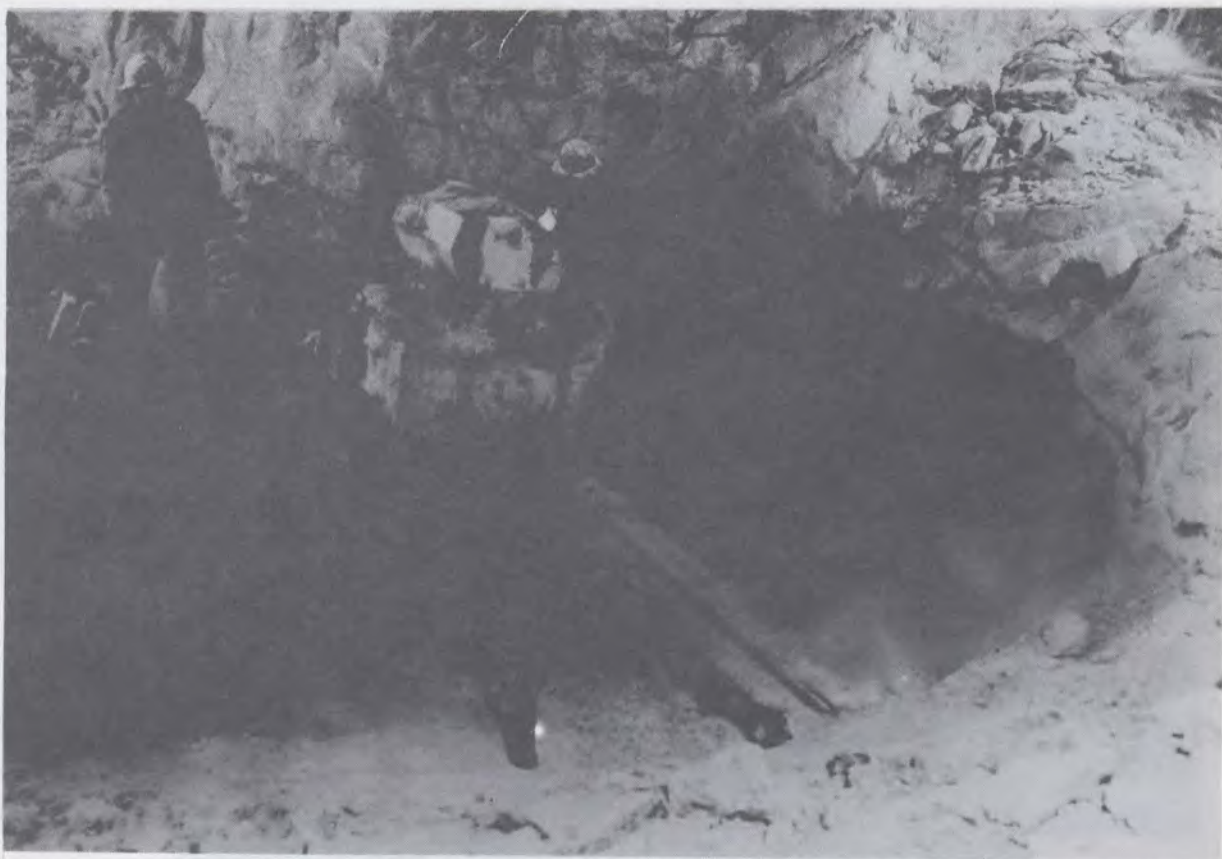
Undercutting face to be blasted, Pugwash Mine (NSIS).
