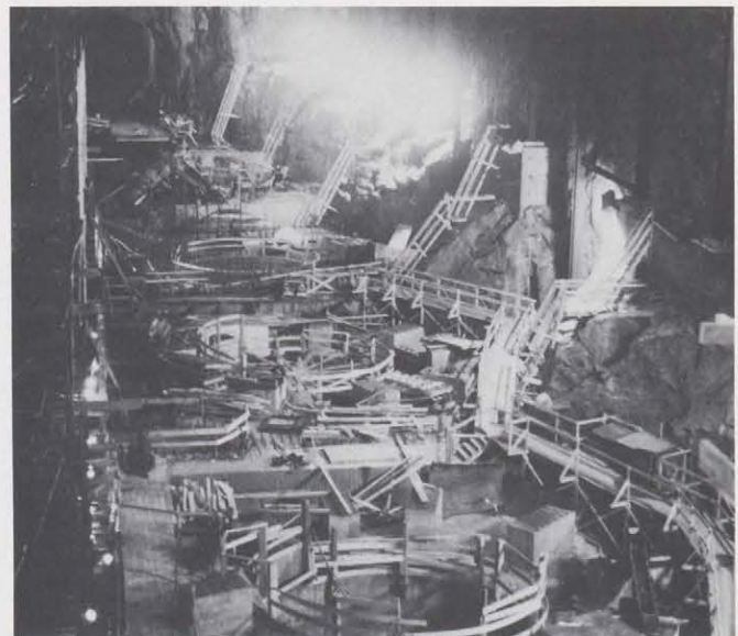
Underground power house construction at the Manicouagan III generating station.
