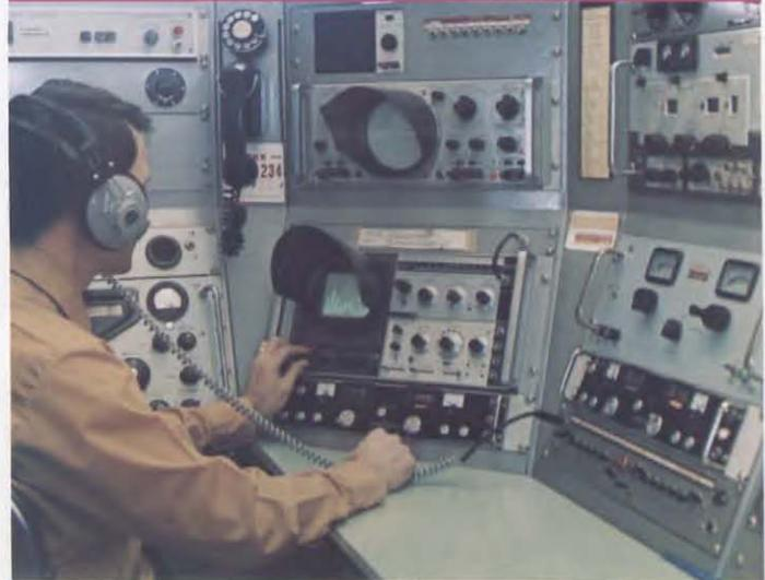
Microwave repeater stations carry nearly all Canada's long distance telephone, data and television traffic. Stationed at line of sight intervals of about 30 miles to avoid interference from physical obstructions, they form some of the longest communications networks of their kind in the world.
