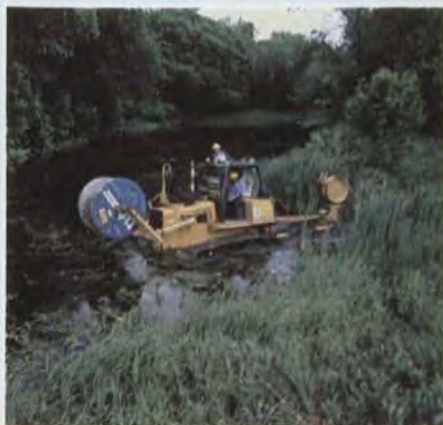
Laying optical fibre
