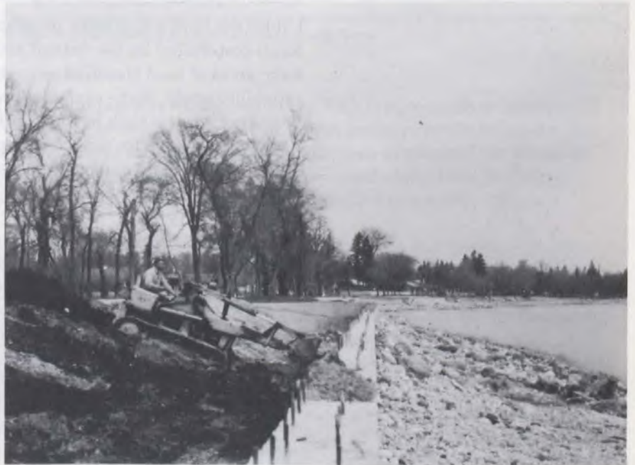
A breakwater was constructed at Winnipeg Beach.
