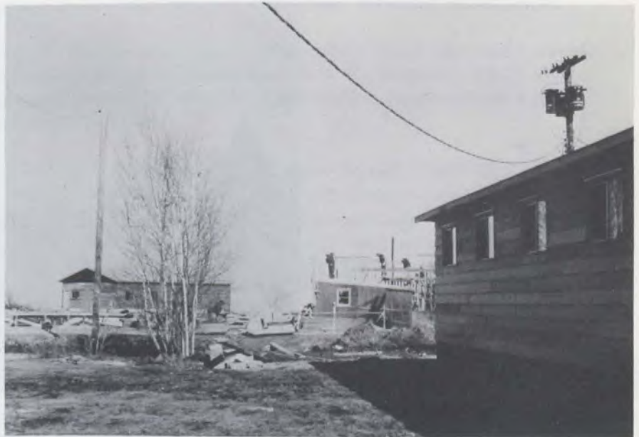
Manitoba Fisheries Training Centre at Hnausa, shown under construction, was Canada's only fresh water fisheries training centre.
