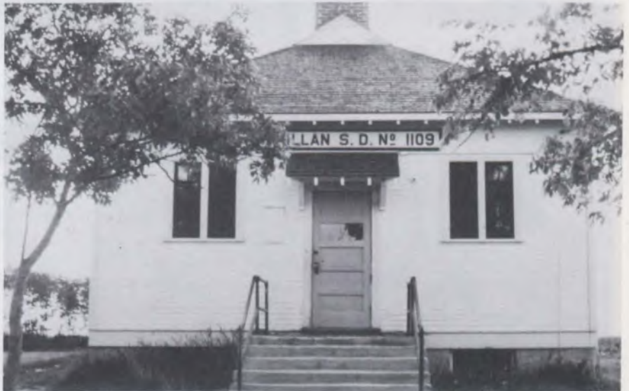
Development under the federal-provincial FRED agreement replaced the many one-room schools in the Interlake region.
