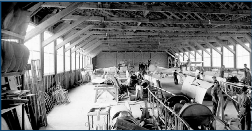
The RFC-C aeroplane repair section at Camp Borden, 1917. Trainee pilots could be very tough on the Curtiss JN-4s. Here, aircraft are in various states of disassembly as they are repaired.
