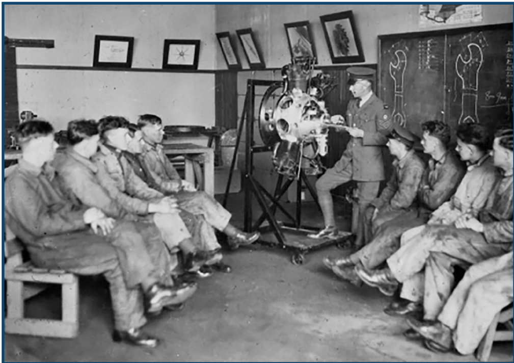
A lecture during the fitter's course, Camp Borden, circa 1932. The airmen instructors passed on not only knowledge about the functioning of aircraft engines but also lessons on field maintenance and repairs learned through experience.
