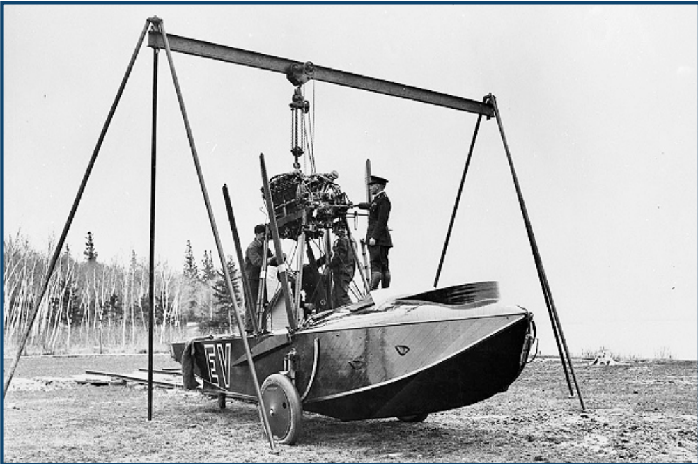
Ground crew change an engine on a Vickers Viking flying boat G-CYEV at Victoria Beach, MB, 15 May 1924. Engine changes could be done without removing the wings, but the necessary equipment to do so in remoter locations did not exist. This type of operation was normal in the field. Reinstallation of the wings was a time consuming process, especially tensioning the rigging to its correct strength.
