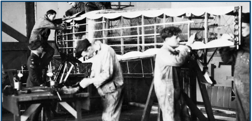
The advanced part of the riggers course involved taking apart and rebuilding static airframes. Here a staff sergeant supervises a group of trainees during the rebuilding process on an airframe at Camp Borden, circa 1932.
