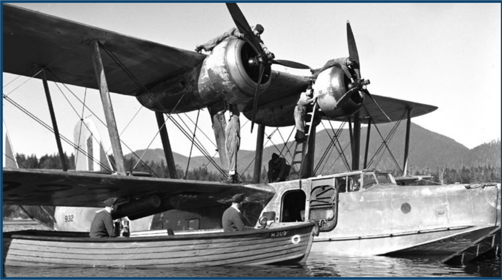
An RCAF marine craft and crew conduct a morning inspection of a Supermarine Stranraer flying boat while maintenance personnel prepare the 4 Squadron aircraft for the day's mission. The RCAF's marine fleet ranged from small rowboats to larger cargo craft.
