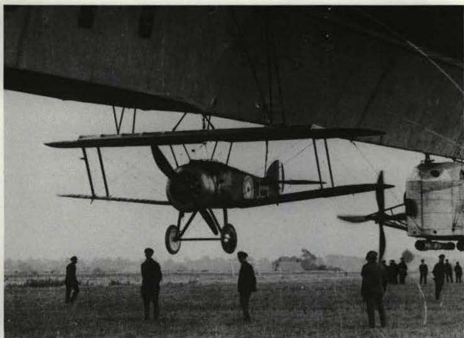
One way to keep fighter aircraft at height in readiness to attempt interceptions of enemy bombers was to suspend them from airships. In a 1918 experiment this Sopwith Camel was slung beneath the R33. (AH 198)
