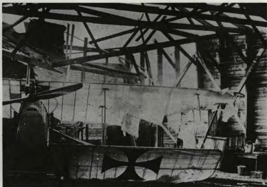
Bomb damage inflicted on a hangar and a German aircraft near Ghent 1917 (Q 109949)
