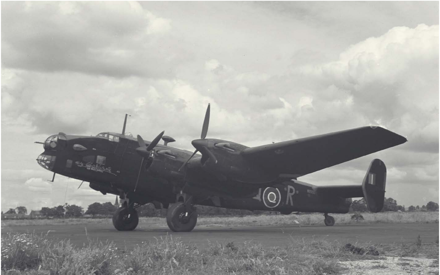
This Halifax B.II aircraft is from 405 "City of Vancouver" Squadron. Coded "LQ-R," this airframe was RAF serial W7710, and it was named "The Ruhr Express" by its crew. Note the Rolls-Royce Merlin engines on this mark. (RCAF photo PL-10458)
