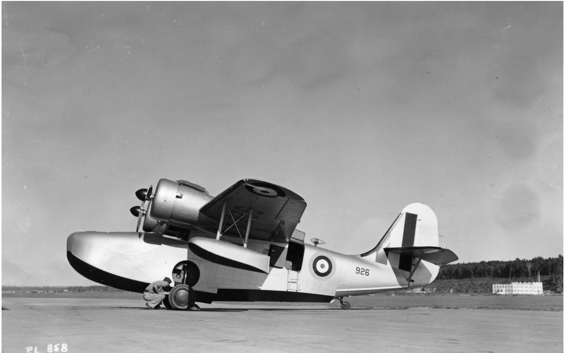
This view shows a pristine-looking RCAF Grumman Goose aircraft on the tarmac at RCAF Station Rockcliffe. Goose 926 was first taken on charge in July 1940, and it first served with No. 121 (K) Squadron at RCAF Station Dartmouth, NS. This aircraft was struck off charge in June 1942 and sold onto the Canadian civil register. Although some RCAF Goose aircraft could be found in camouflage colours, many of these aircraft were finished in a plain, silver paint scheme similar to that illustrated here. (RCAF photo PL-858)
