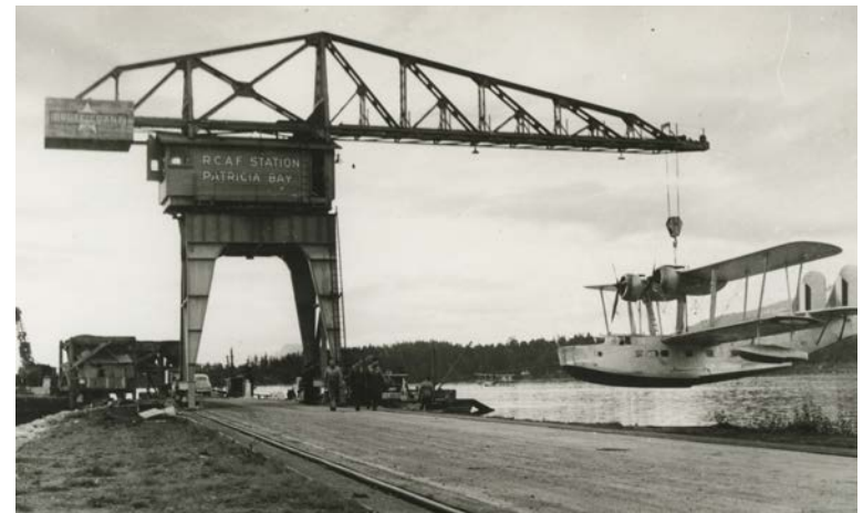
The Stranraer was pure flying boat and consequently it needed cranes or beaching gear to be brought onto land. This heavy-lift gantry crane was part of the facility at RCAF Patricia Bay, BC. (RCAF photo - CY22-7-GL)
