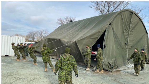
2 - Dismantling of a MEX-26 shelter by the mission closure team at Mihail Kogălniceanu Air Base, Romania
