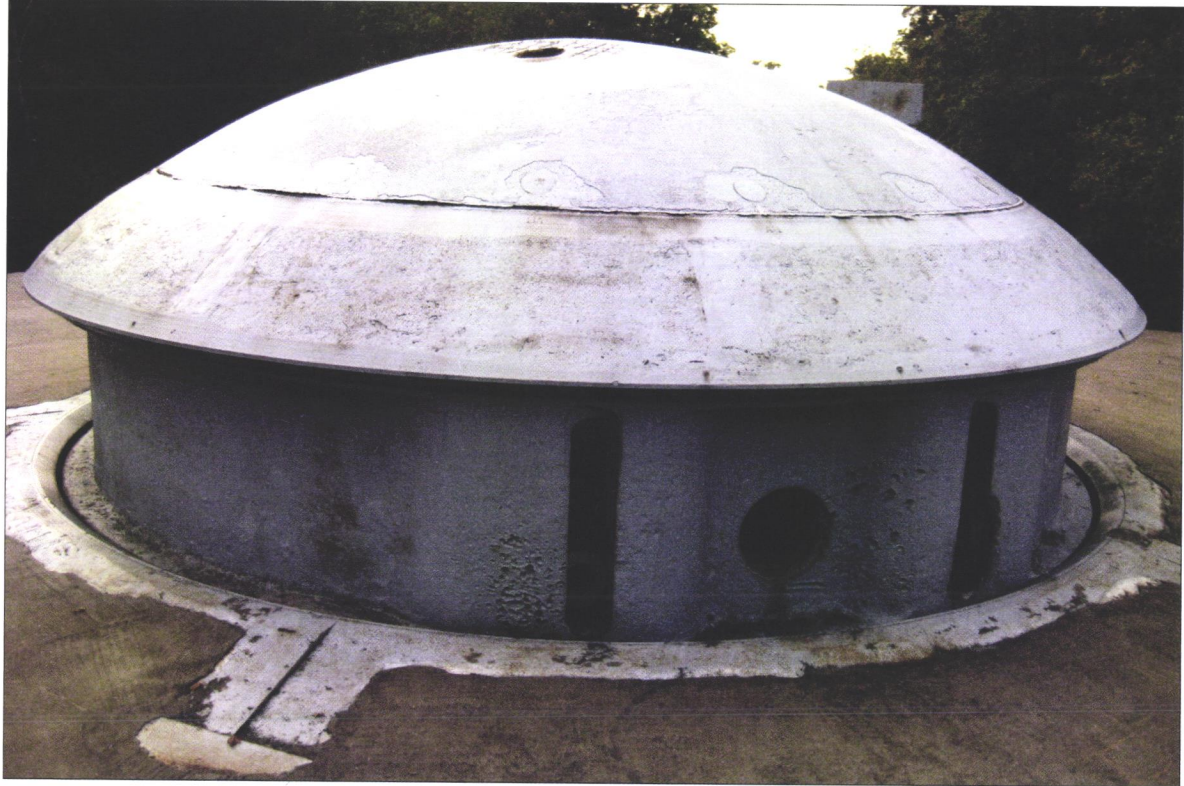
Retractable, rotating cupola with 75mm guns.
