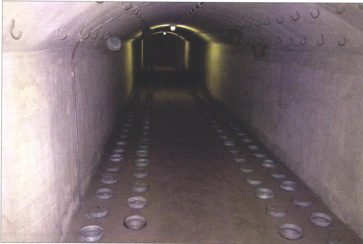
Corridor with protective equipment against gas attack.
