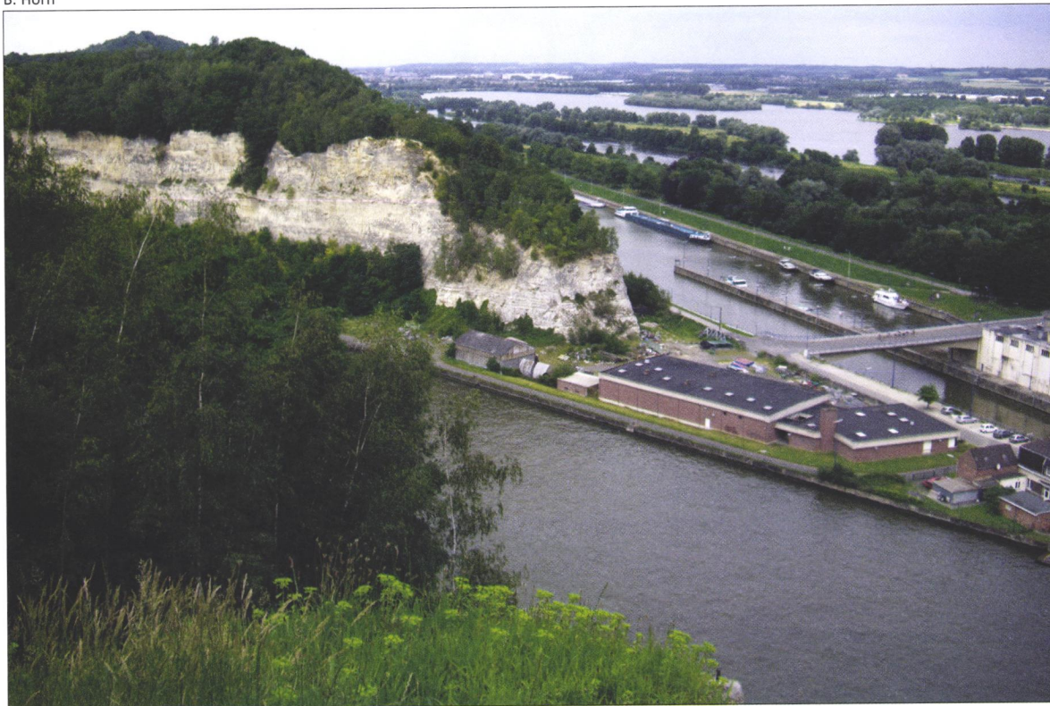
The cutting of the Albert Canal at Caestert, 2012.
