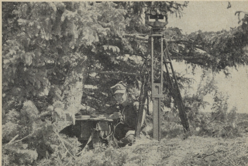
A radar listening post showing the flash spotting instrument with remote control to a No. 52 radio set.
