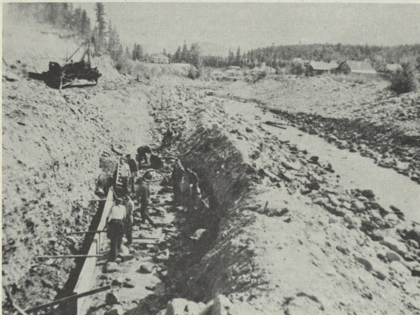
The pier excavation for the Mark Creek project.
