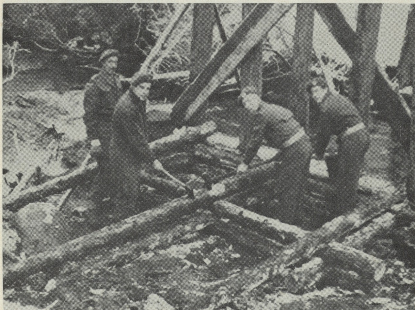
Cutting timbers for the pier crib.
