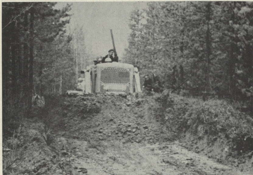
Bulldozing the road to Cherry Creek site.
