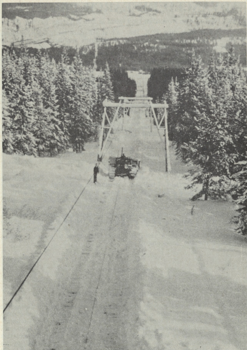
Stringing the tee-bar tow cable.
