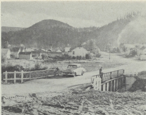
The new bridge completed and open to traffic.
