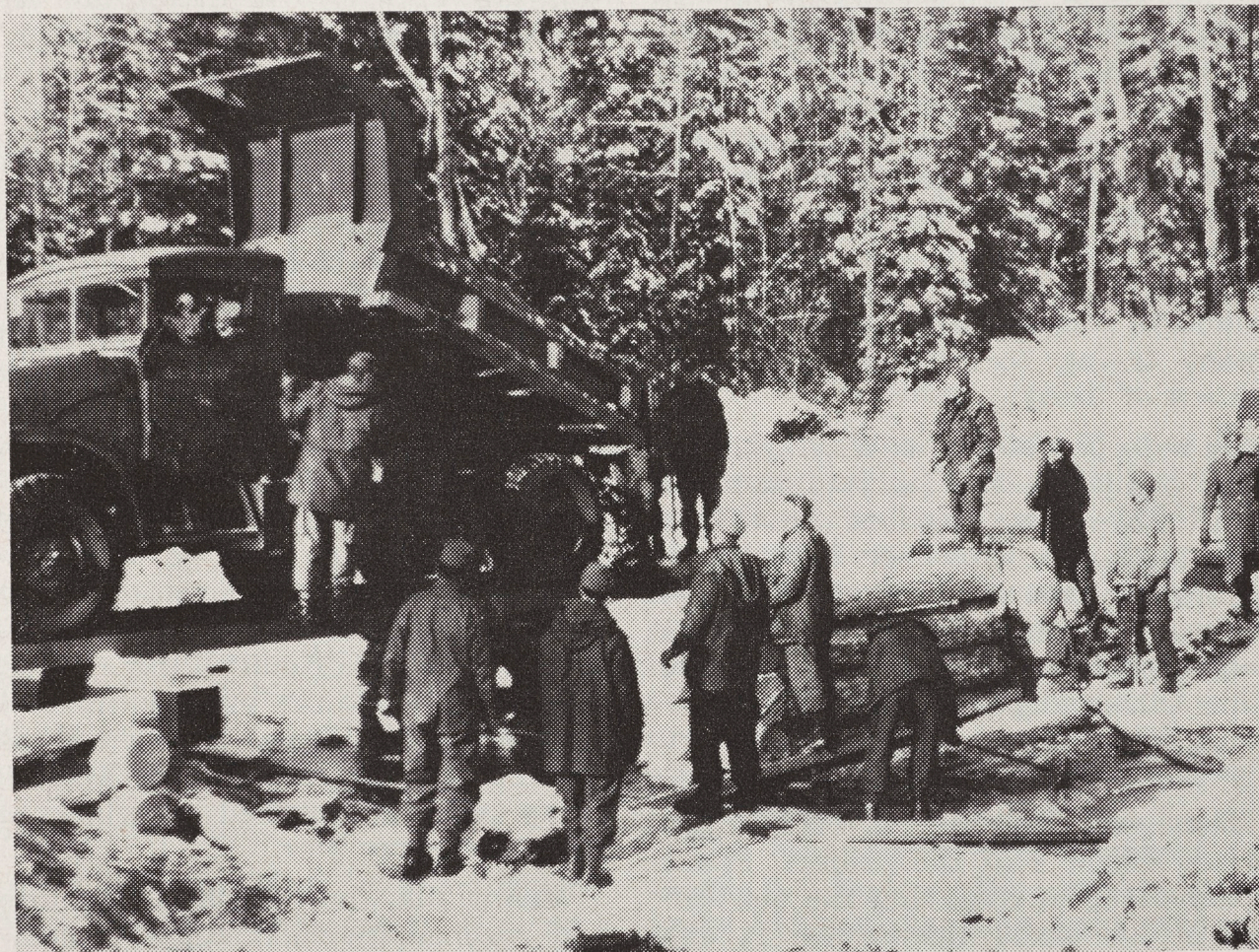
Filling the centre crib pier with gravel.
