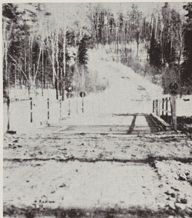
The completed bridge. Note the steep hill in the background.
