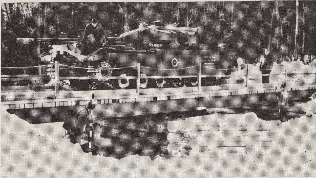
Stresses are checked while a Centurion tank is on the bridge.
