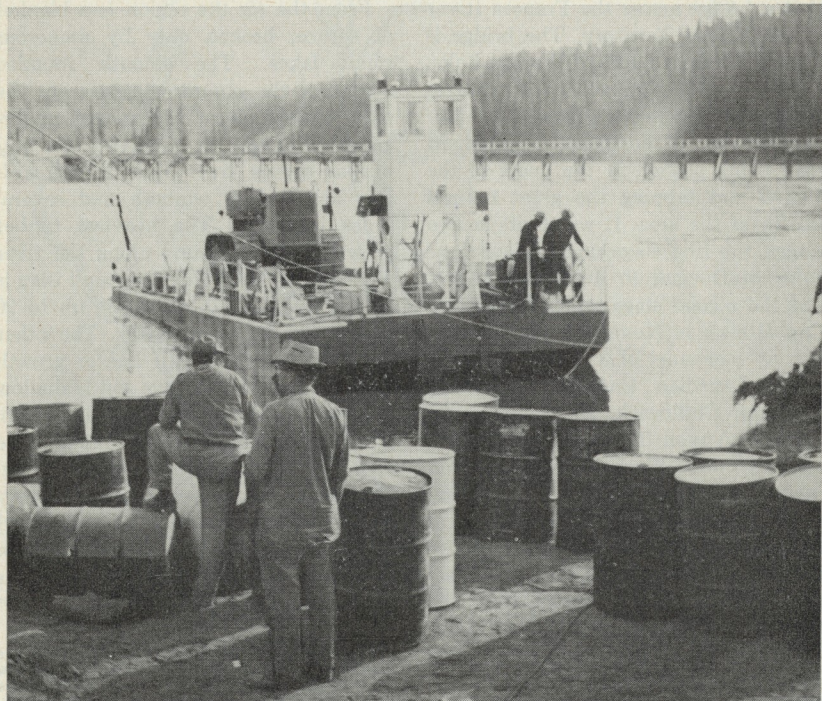
A barge loading at Mile 36 (lower end). This was to have been used to move equipment to the construction site, but when the river level dropped, plans had to be changed. The bridge in the background is the temporary Lower Frances River bridge.
