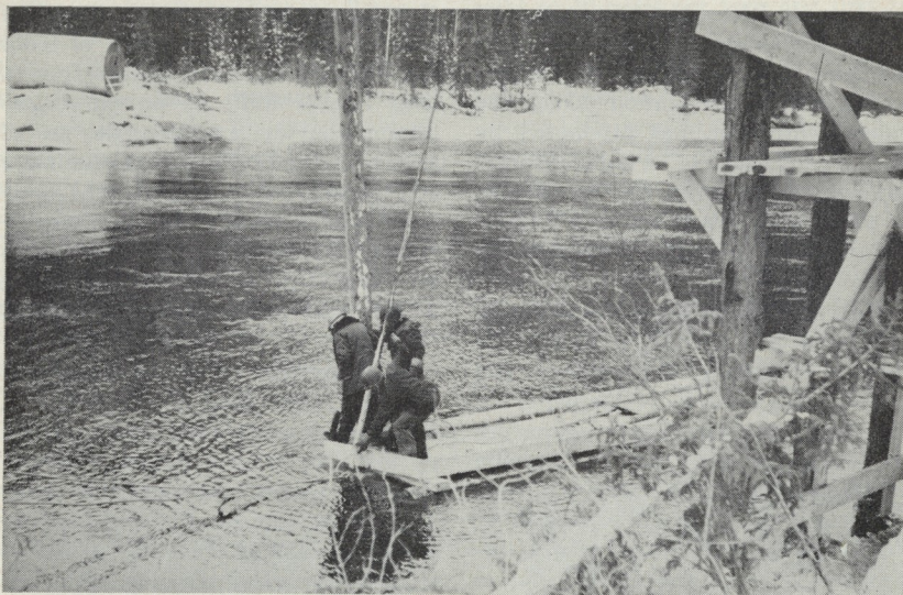
A small raft is used to guide the piles.
