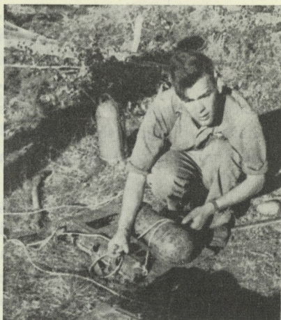
The Wild T-2 transit being strapped to a packboard.
