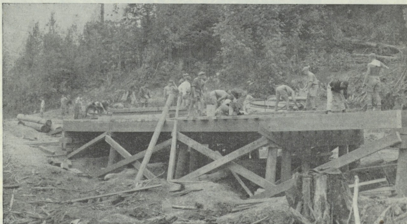
A close-up of the partially-completed bridge.
