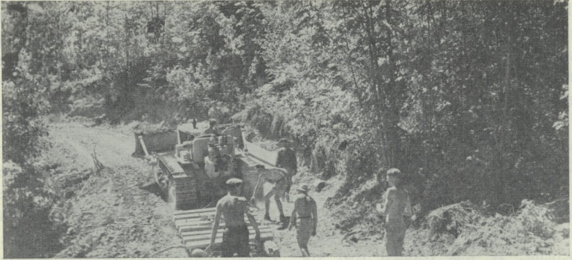
Widening the road with a bulldozer.
