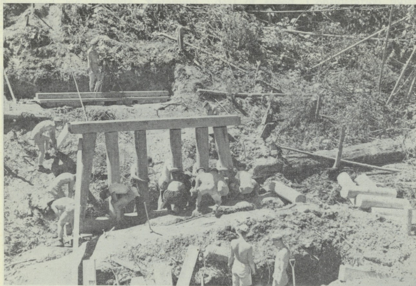
Erecting the supports for the single bent trestle bridge.
