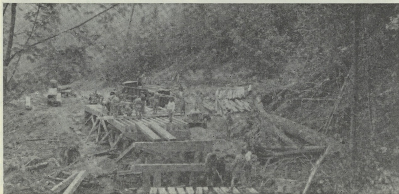
Another view of the bridge under construction.
