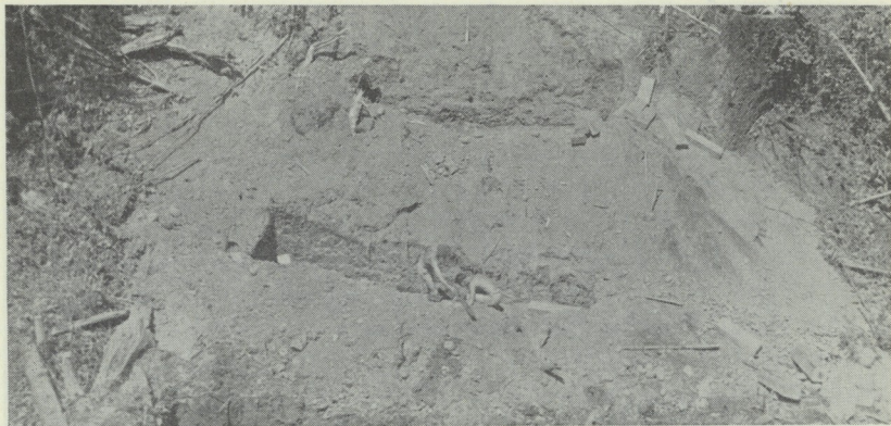
Excavating for the bridge footings.
