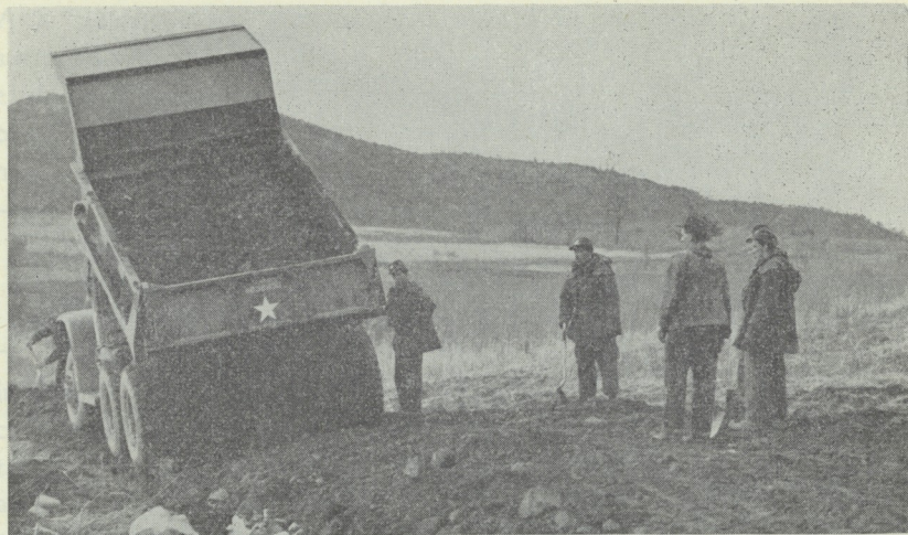
Above: A dump truck unloads loose fill for surface dressing on a new road. Below: A bulldozer pushes through a road over rugged country in Korea.
