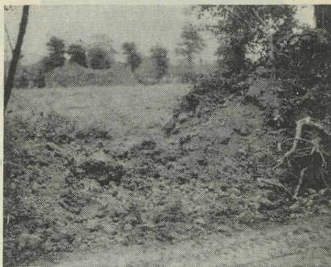
Hole cut through a thick hedgerow by blades mounted on tanks.
