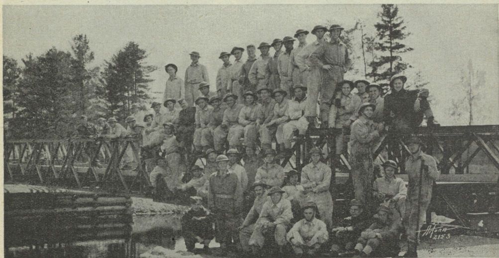
A Bailey bridge built by the McGill University Contingent, COTC, at Petawawa Camp in 1945.
