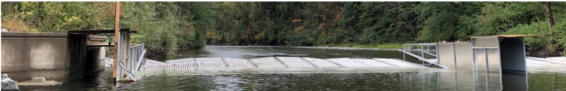
Figure 2: Two-passage counting fence configuration with wide passageways located mid-river and at the bulkhead, first piloted in 2019.
