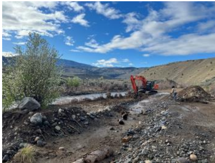
Figure 1: Excavator constructing a low bench.
