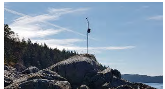
Image 1: Weather station installed at remote site. Credit: Glenn Cooper (Fisheries and Oceans Canada)
