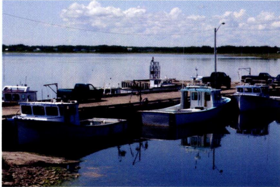
Inkerman's wharf, a provincial harbour located in the Acadian Peninsula.
