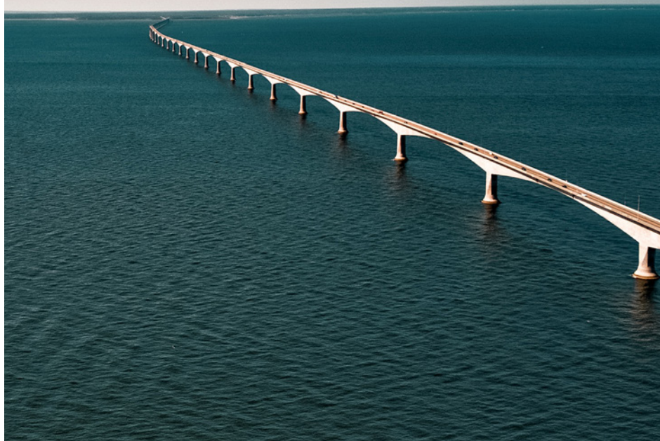
Bridge to Prince Edward Island. Mkdroner. Unsplash.
