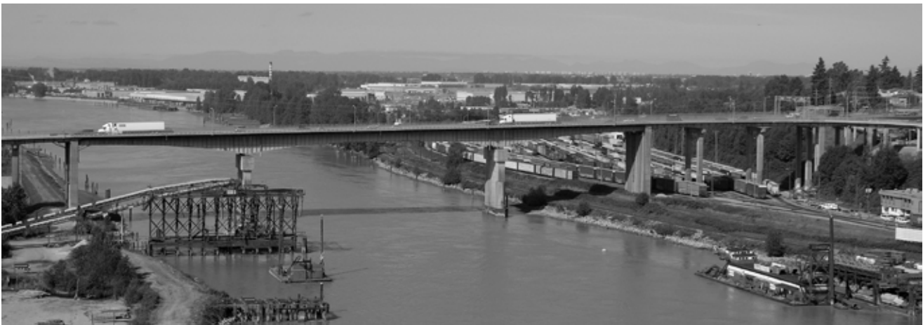
QUEENSBOROUGH HIGHWAY BRIDGE (2007)
