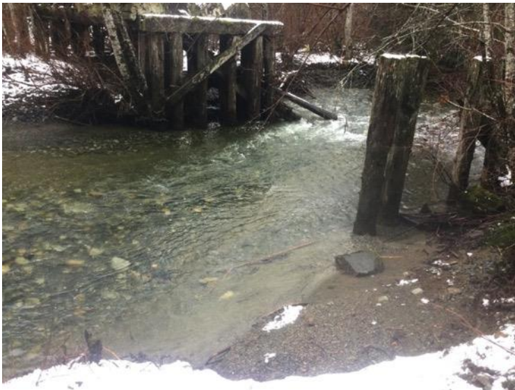
3.) North Nanaimo overflows left bank to 590m channel
