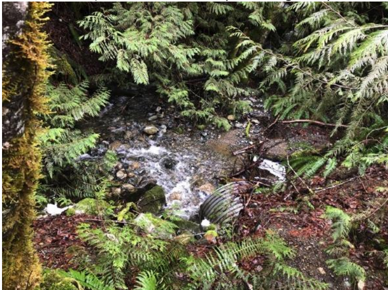
3.) R13 Placemark 9 culvert under rail grade
