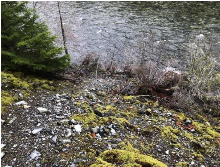
5.) R12- Slide track along rail grade needs planting
