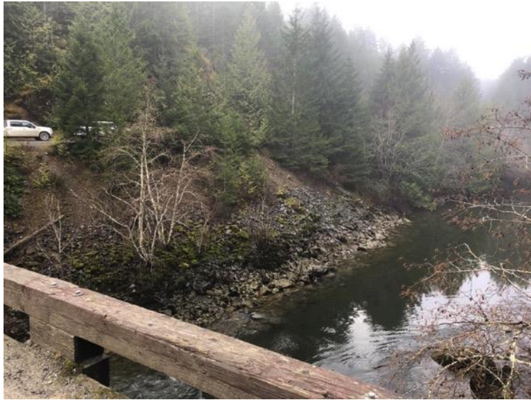
1.) Spawning Gravel placement – possible access site.
