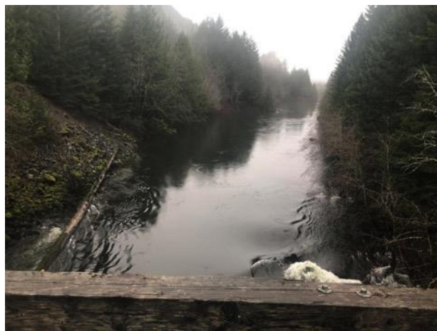
Reach 16 has 80m armoured bank at bridge.
