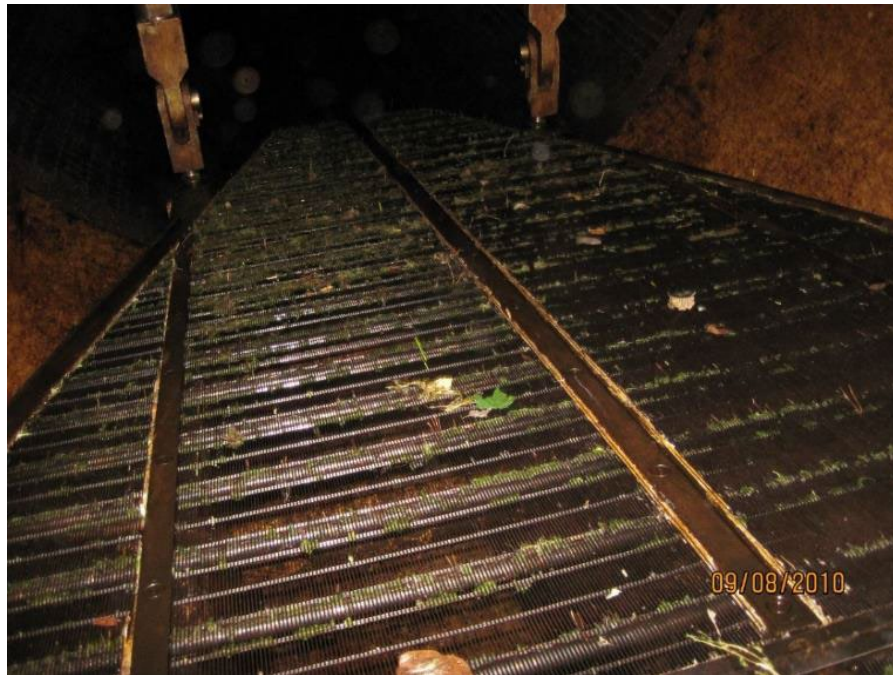
Figure 83. Top of the upstream end of the Eicher Screen. This section of screen is typically cleaner than the rest of the screen (Photo: Sheng 2010).
