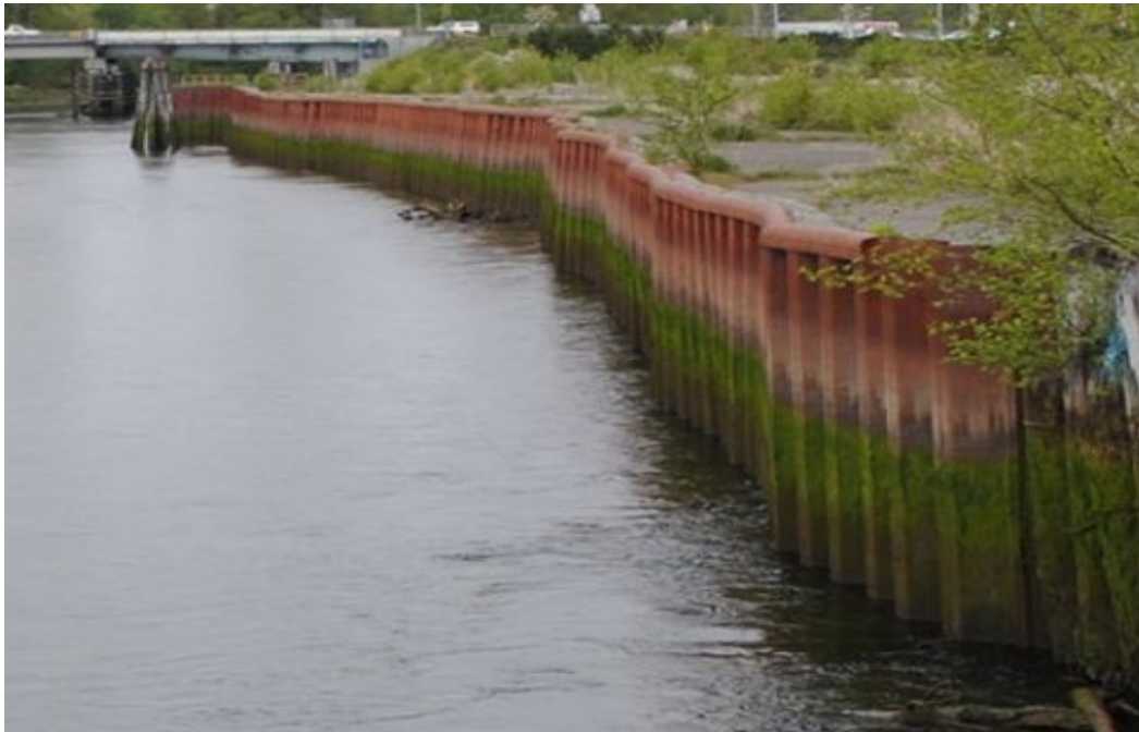
Figure 41. Steel-clad concrete retaining wall along the site (Source: Project Watershed).
