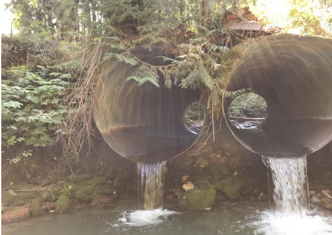
Figure 1. Example of barrier culvert on Chuck Creek, BC.
