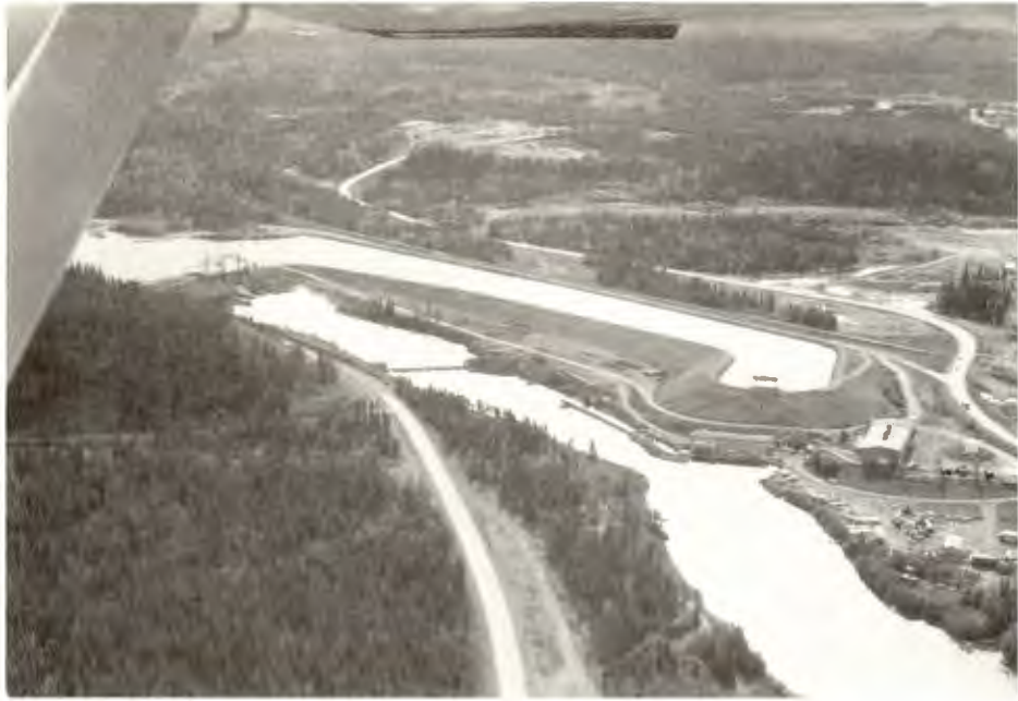
PLATE 1: Whitehorse Rapids hydro-electric power development
