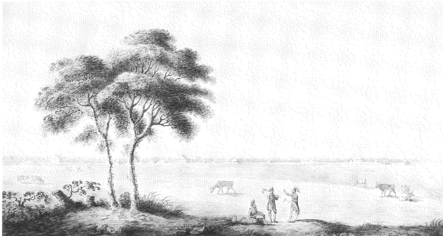
23 View of Île aux Noix at the end of the 18th century; two blockhouses built in 1776 can be seen. (NA, C-40335)
