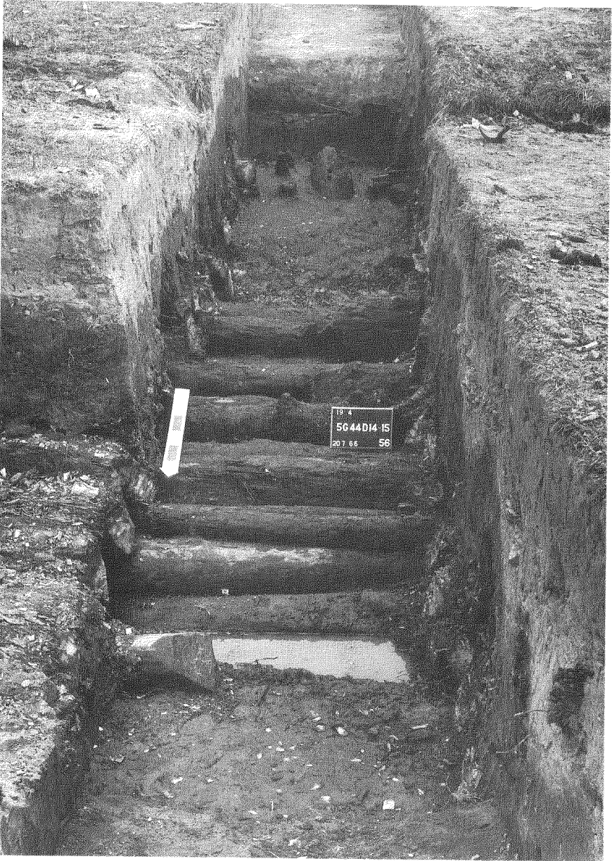
51 Wooden logs found in the ditch of the north face of the first British fort. These pieces belong to the original revetment of the escarp. ( Parks Canada, R.T. Grange, Jr., 5G44: 19Y6 )
