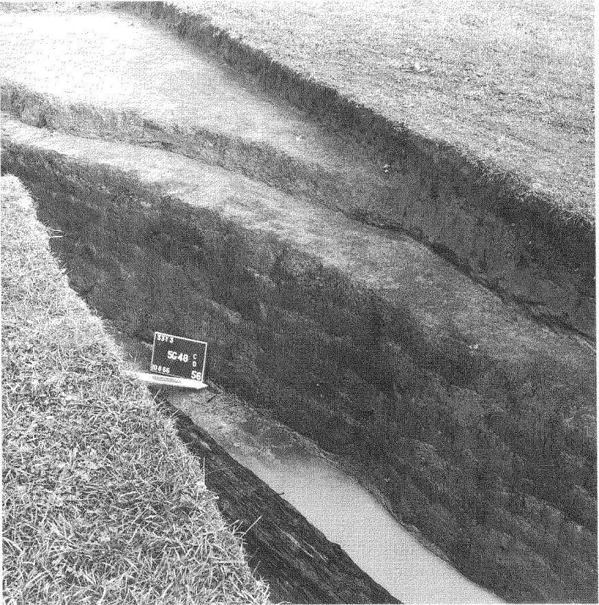
28 Sodded revetment of the northwest corner of the counterscarp, excavated in 1966. ( Parks Canada, R.T. Grange, Jr., 5G48, C, D: 33Y3 )
