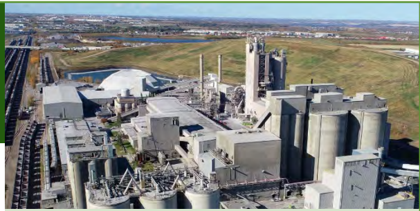
Heidelberg Materials' cement plant in Edmonton, AB – Heidelberg Materials
