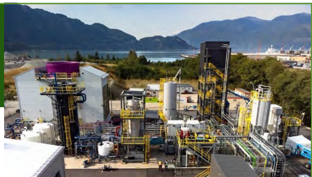
Carbon Engineering's Innovation Centre in Squamish, BC – Carbon Engineering
