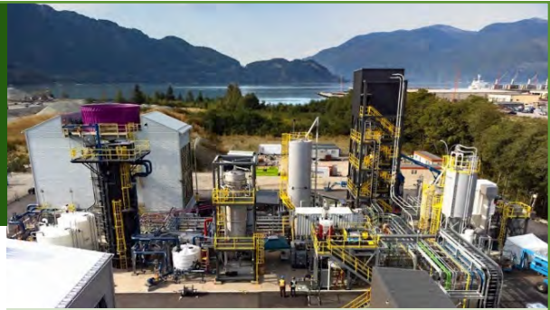
Centre d'innovation de Carbon Engineering à Squamish, C.-B. – Carbon Engineering
