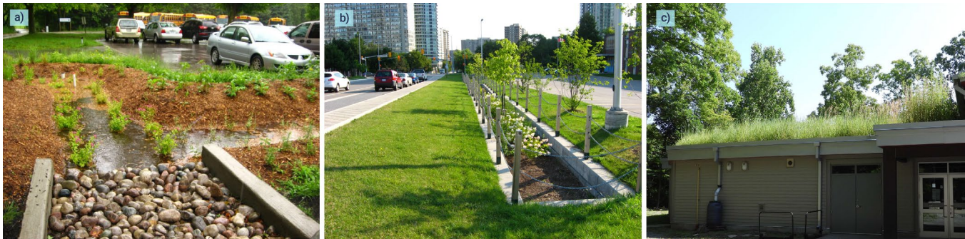
Figure 5: Images of different nature-based approaches for addressing stormwater runoff: a) Parking lot of the Kortright Centre in Vaughan, Ontario with integrated bioretention (photo courtesy of Daniel Philippi, 2022); b) Bioswale along Elm Drive in Mississauga, Ontario (photo courtesy of Daniel Philippi, 2022); and c) Green roof on the District School Board of Niagara's Walker Living Campus at the Woodend Conservation Area, Ontario (photo courtesy of Jocelyn Baker, 2023).
