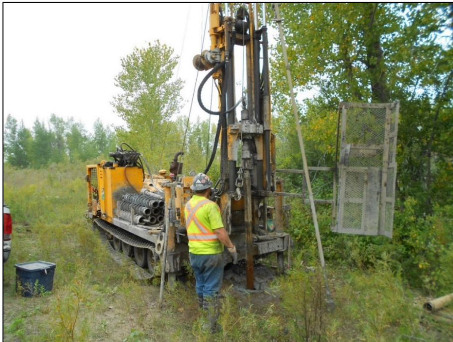
Figure 7: Drilling of the stratigraphic borehole by casing advancement. Photograph by J.B. Percival. NRCan Photo Database number 2020-638.
