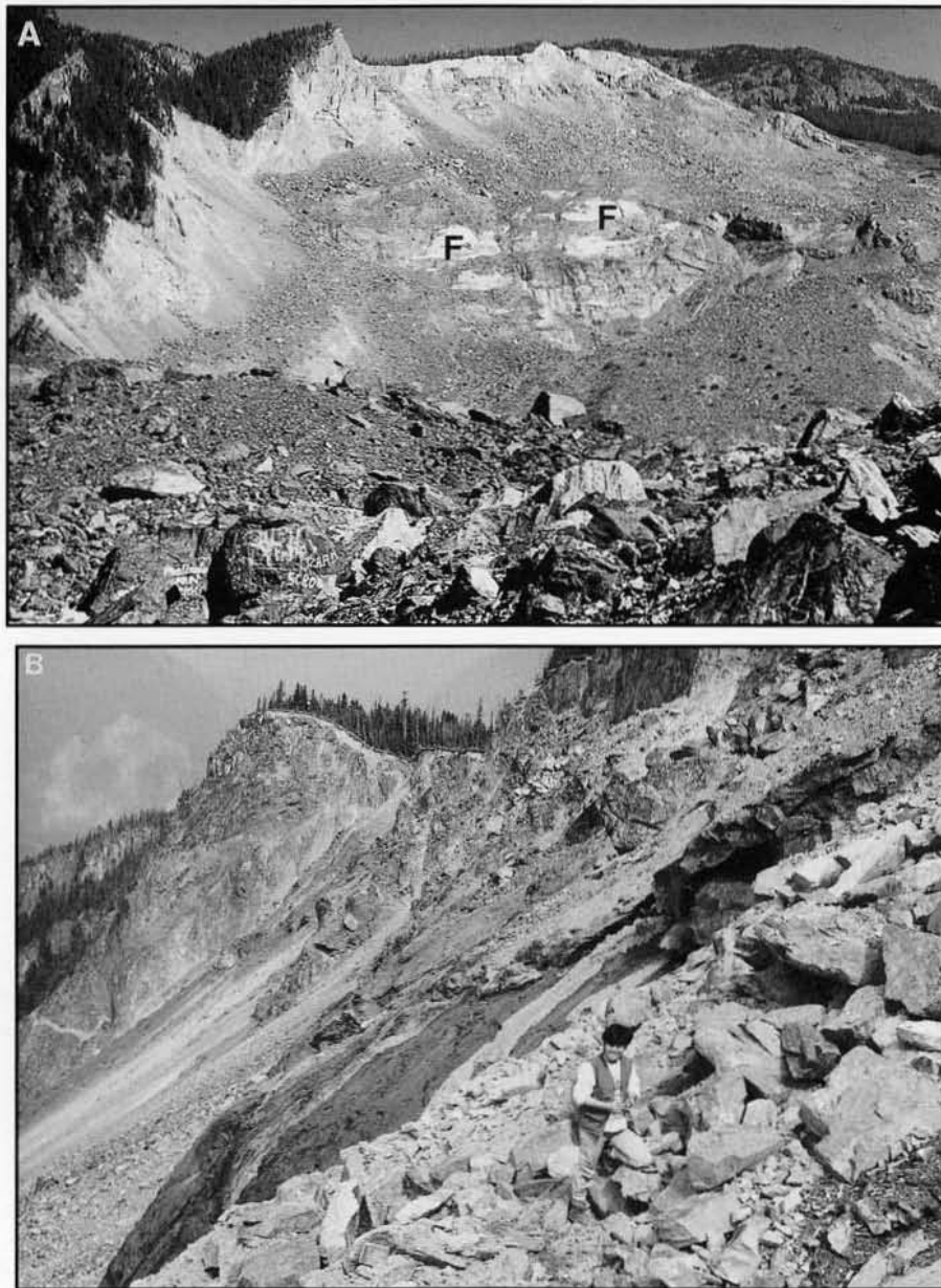
Figure 11. A) 1965 Hope Slide sliding surface and debris; felsite sheets (F) in lower part of the slope. GSC 1994-738 B) Sliding surface in upper part of the slope. Note steep irregular surfaces in greenstone. GSC 1992-114B
