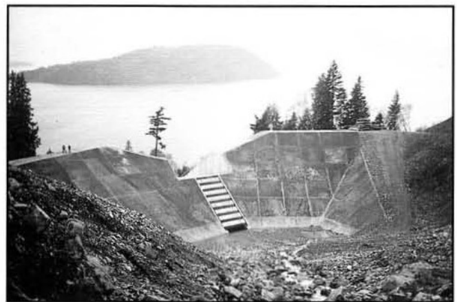
Figure 38. Debris flow retention structure on Charles Creek, Howe Sound constructed in the mid-1980s; view downstream. GSC 1991-298
