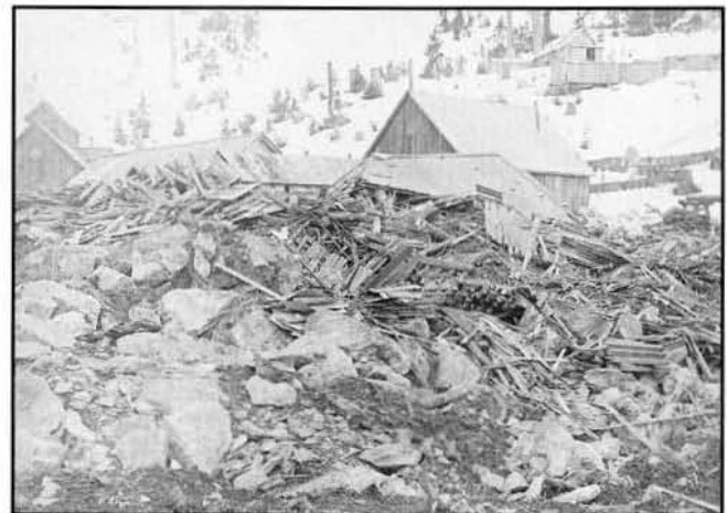
Figure 9. Destroyed buildings and rock debris at Jane Camp, Britannia mine, following the 1915 rock avalanche which resulted in 56 deaths. The Jane Camp tragedy is Canada's second largest landslide disaster, after the 1903 Frank Slide (photo by British Columbia Museum of Mining).
