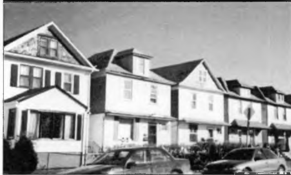
Foursquare house with mansard roof and rectangular house with hip roof
