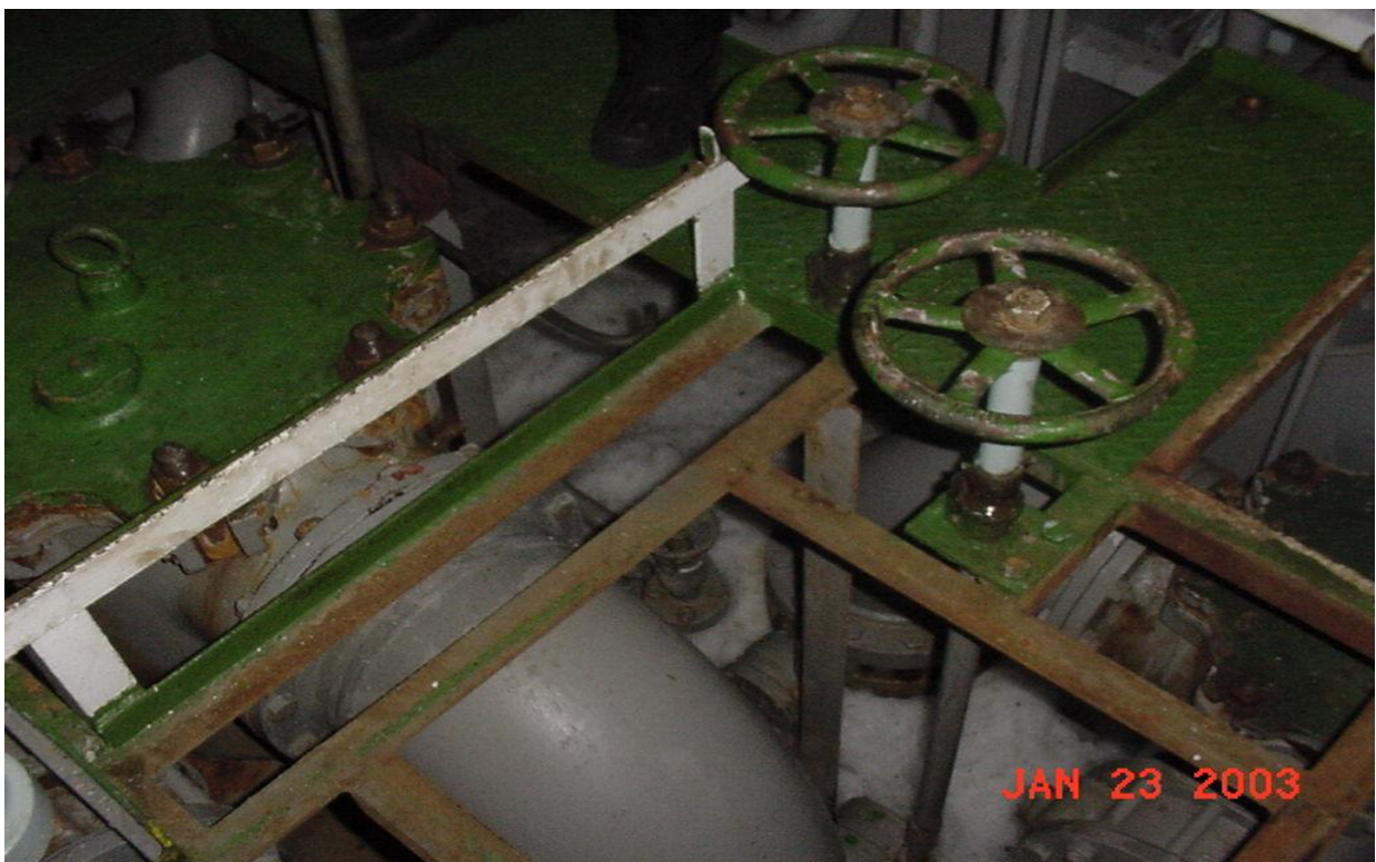
Figures 3.7B – Frazil ice accumulation in bilges due to strainer cleaning
