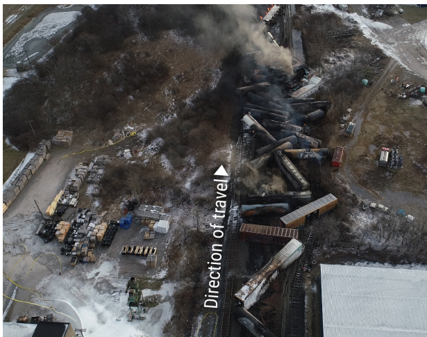
Aerial photograph of derailment site in East Palestine, Ohio. Courtesy: National Transportation Safety Board (NTSB)
