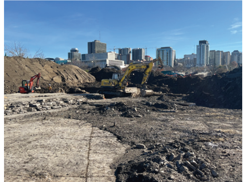
Remediation work at Victoria Island
