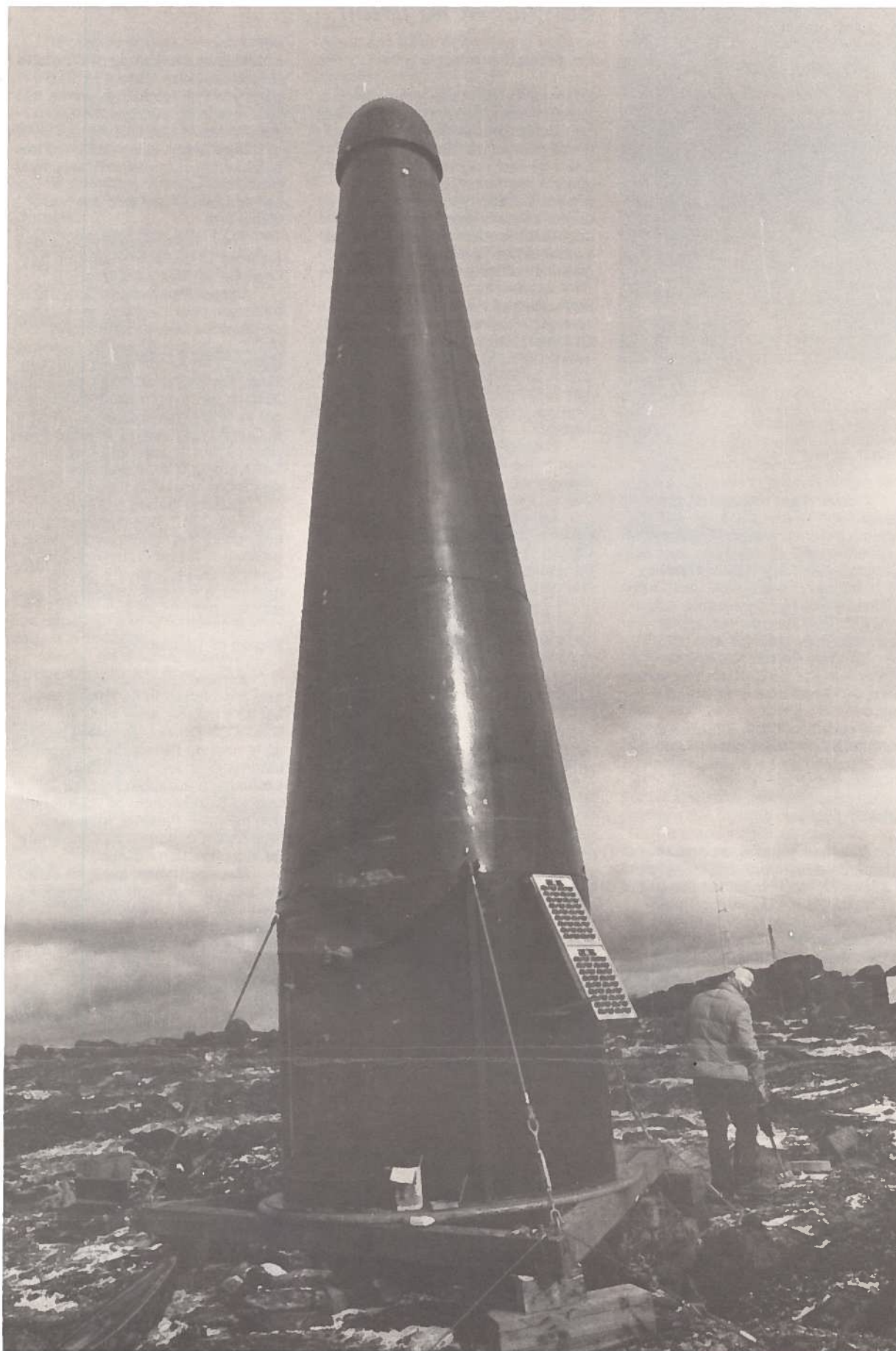
The Comshell is in place. The 24-volt solar panel is used for trickle charging high-capacity lead acid batteries. A technician is drilling holes for rock anchors.
