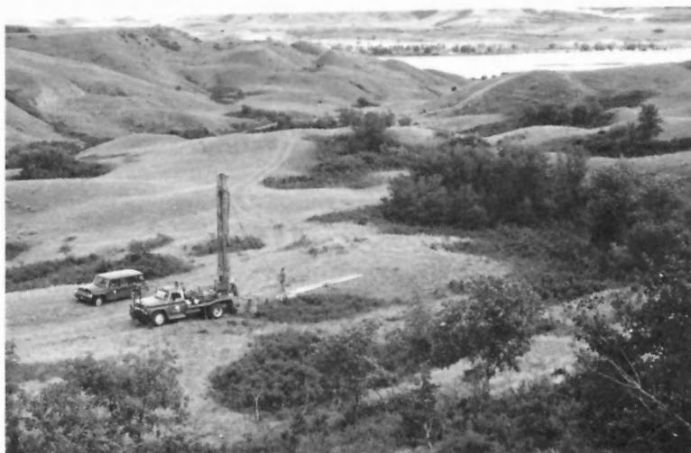
Figure 2. Installation of piezometers in landslide area along stream valley tributary to South Saskatchewan River.
