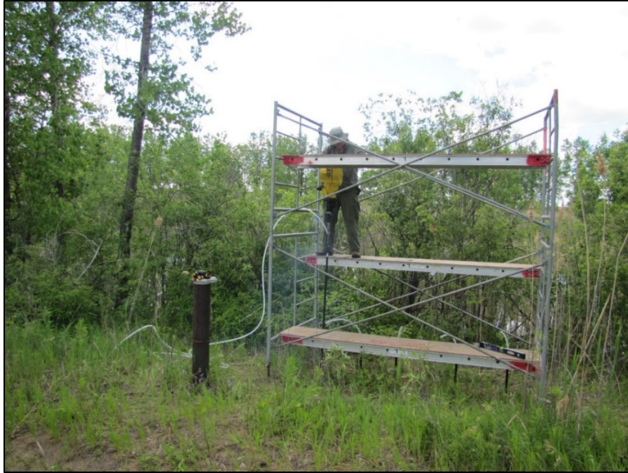
Figure 6: Installation of drive-point piezometers at the study site. Photograph by J.B. Percival. NRCan Photo Database number 2020-635.
