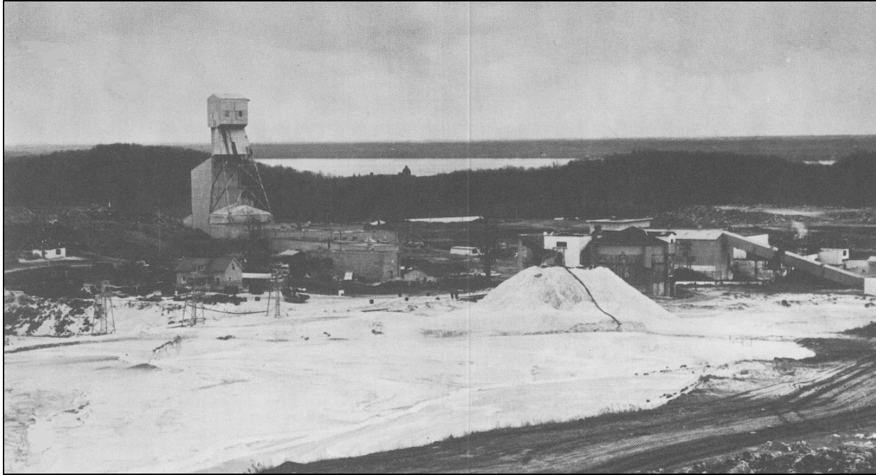
Figure 1: View of the mine site in 1967, looking south toward the Lac des Deux Montagnes. The photograph shows the newly completed headframe and the tailings disposal area in the foreground. Photograph from SLC (1967).
