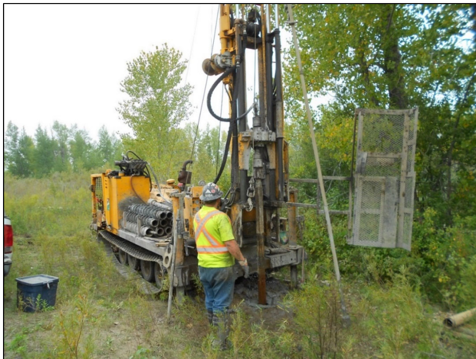
Figure 9: Drilling of the stratigraphic borehole by casing advancement. Photograph by J.B. Percival. NRCan Photo Database number 2020-638.
