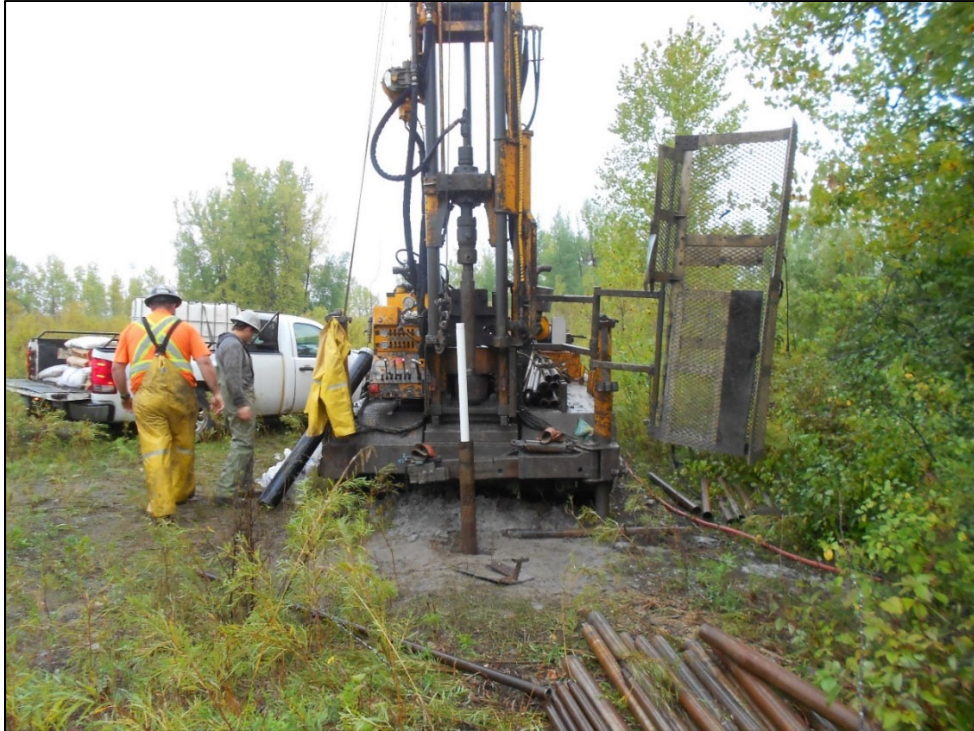
Figure 10: Completion of the stratigraphic borehole as observation well OW-01-G. Photograph by J.B. Percival. NRCan Photo Database number 2020-639.
