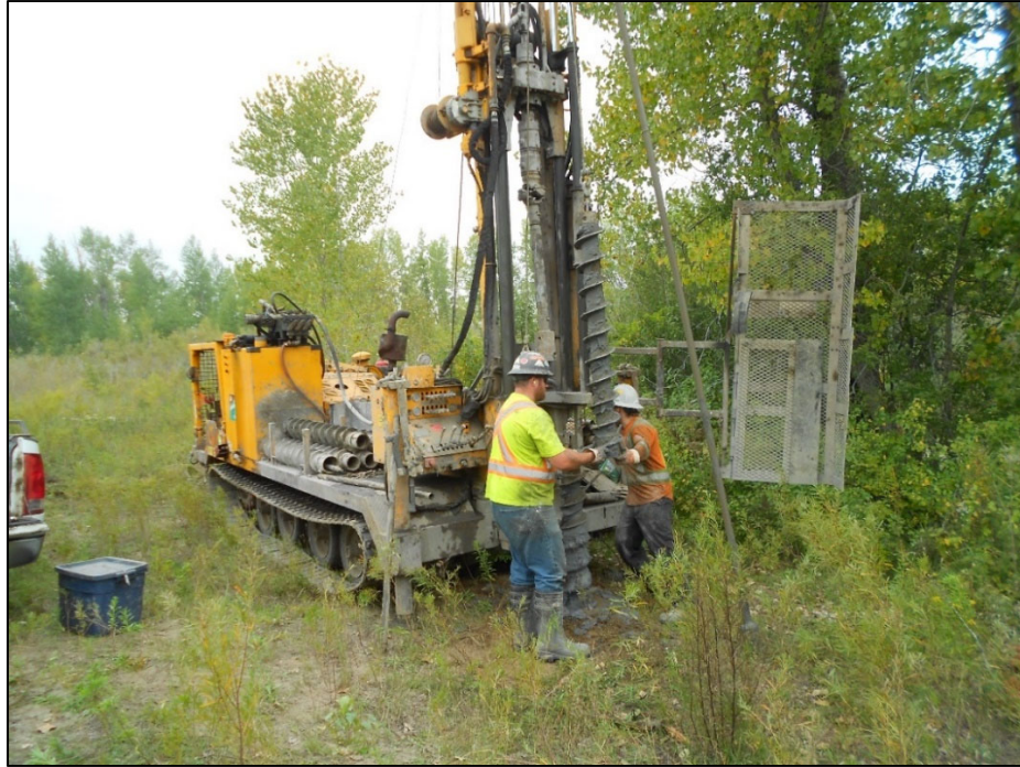
Figure 8: Drilling of the stratigraphic borehole by hollow-stem augering. Photograph by J.B. Percival. NRCan Photo Database number 2020-637.
