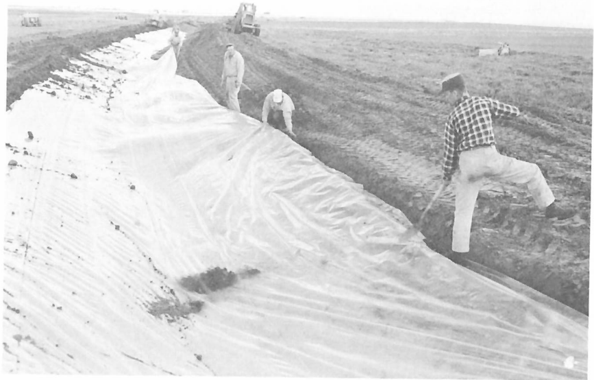
FIG. 8 Installing plastic lining.
