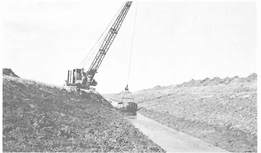
FIG. 10 Open-channel drain constructed by dragline. Note the salt deposits and water-table line on the right side.
