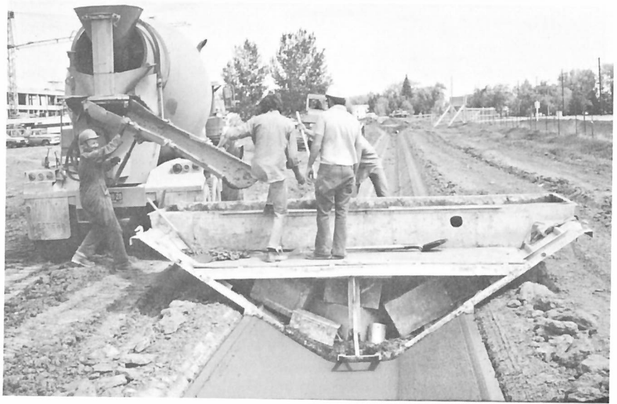
FIG. 7 Slip form used to install concrete lining.
