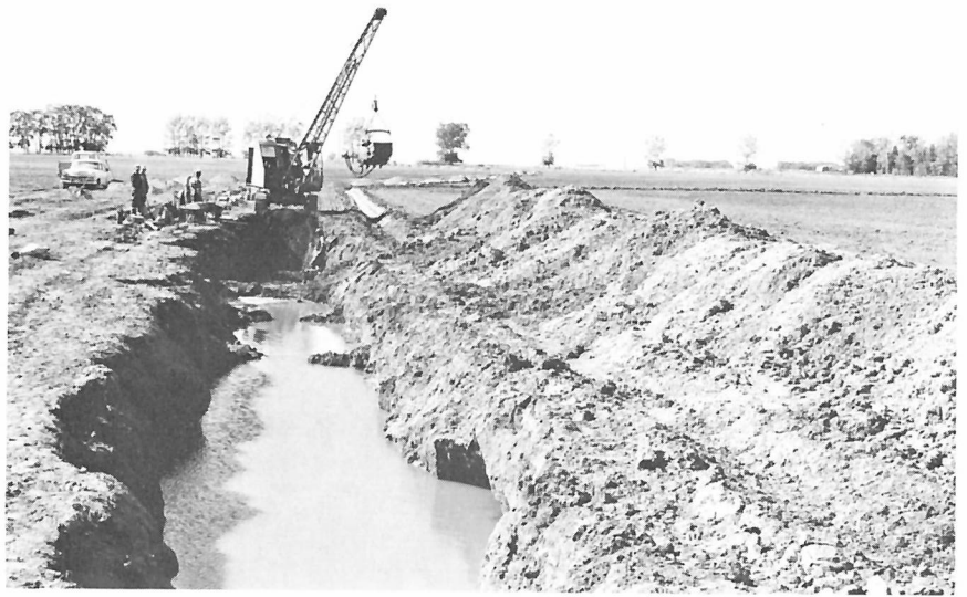
FIG. 17 A dragline is used to lay tile drain under adverse conditions.
