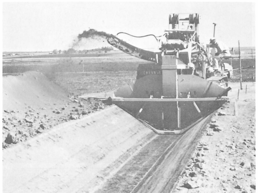
FIG. 6 Rotary excavator used for excavating and shaping the canal to prepare it for concrete lining.
