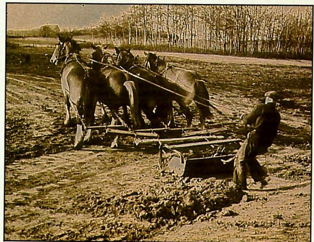
With only a horse-drawn scraper, excavating a dugout was a difficult task.
