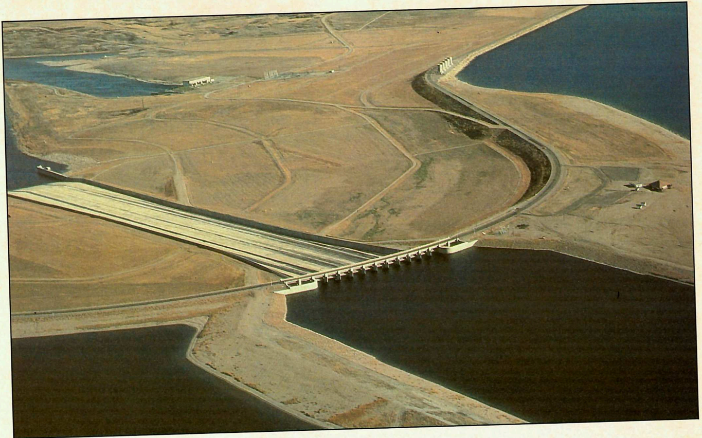
Gardiner Dam. The spillway is shown in the centre, while the hydroelectric station can be seen in the upper half of the photo.
