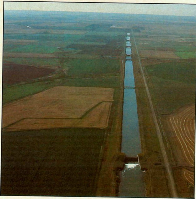
Main canal of the St. Mary Irrigation Project near the town of Taber, Alberta.
