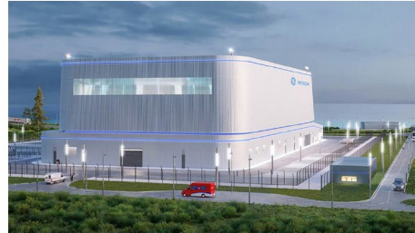
Darlington New Nuclear Project, Clarington, Ontario
