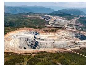
Red Chris Mine Expansion, Northwestern British Columbia
