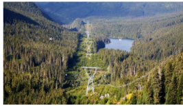
North Coast Transmission Line, Northwest British Columbia
