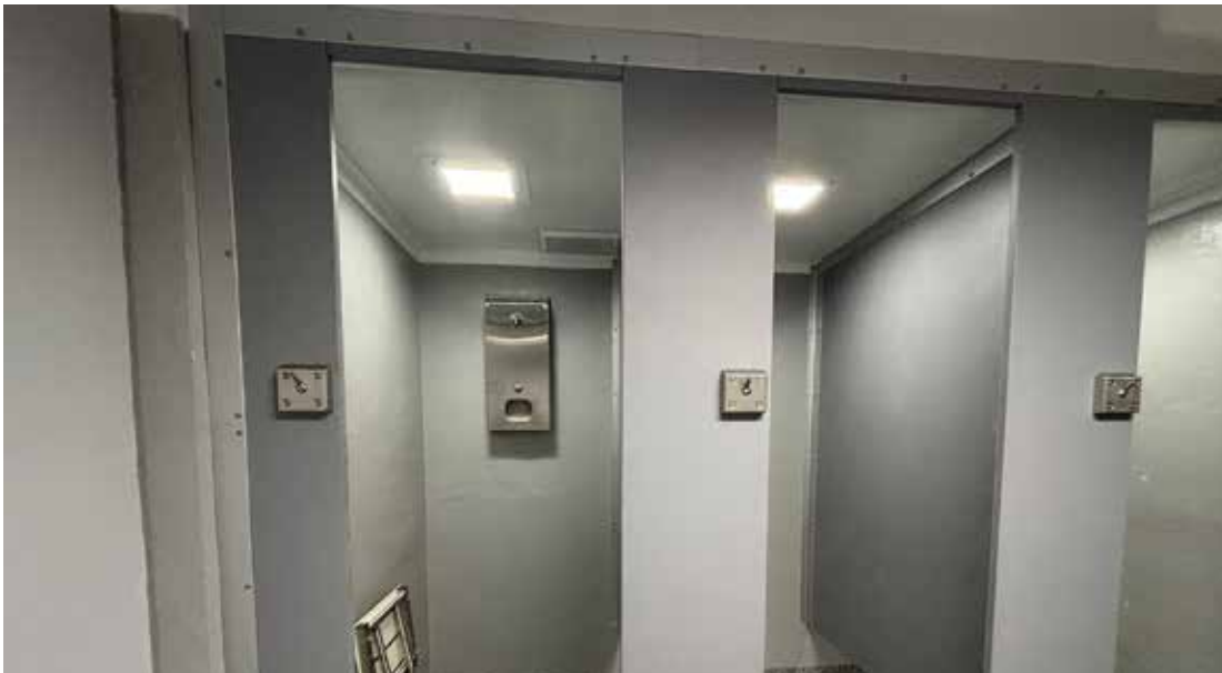
Cowansville Institution, QC - Collapsible shower hooks and a shower head designed to prevent ligature use
