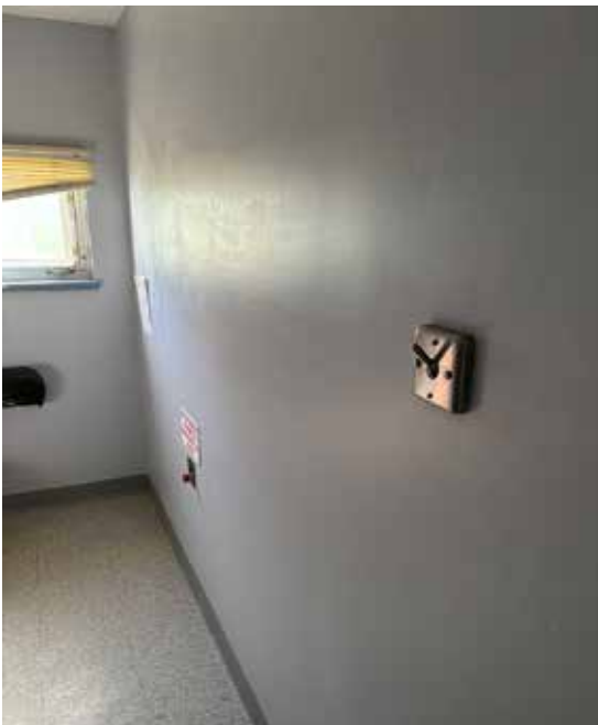
Nova Institution, NS - Collapsible hook designed to prevent ligature use
