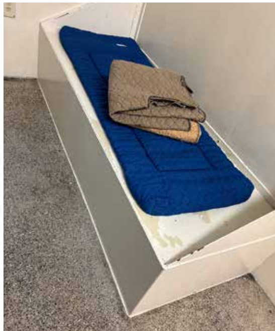
Kent Institution, BC - Bed with a sheet metal frame
