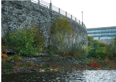
600+ different structures (e.g. retaining walls, lookout platforms, dams and so on)
