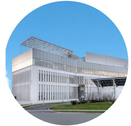
Advanced materials research facility in Mississauga
