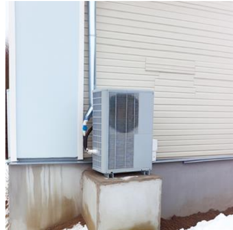
Figure 5. This image shows an exterior view of an example CC-MSHP. Credit: NRC.
