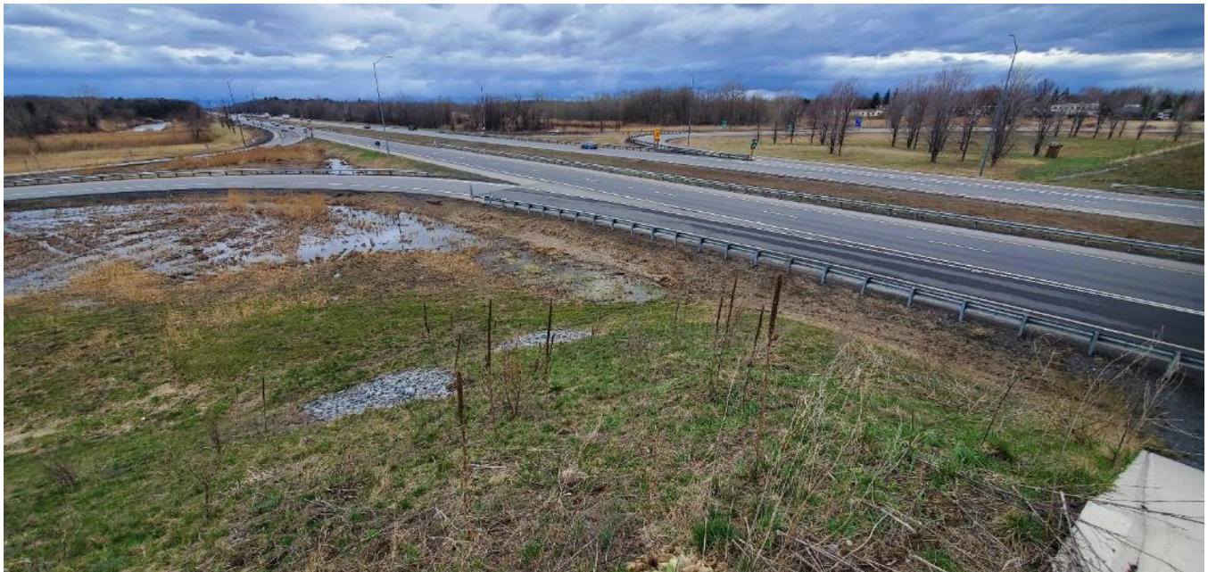
Figure 5-15. Panoramic view of the Highway 401 entry ramp and main corridor from the monitoring site.
