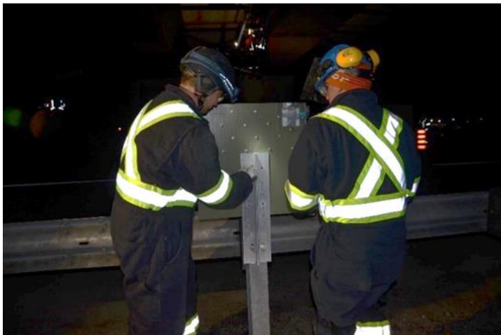
Figure 5-19. Final commissioning of the key system components. Top left: installation of Plate 1 on the abutment wall along with the integrated T/RH sensor; Top right: deployment of the solar panel array on the embankment. Bottom left: mounting of the WS mass-loss specimen holder on the side rail's post.
