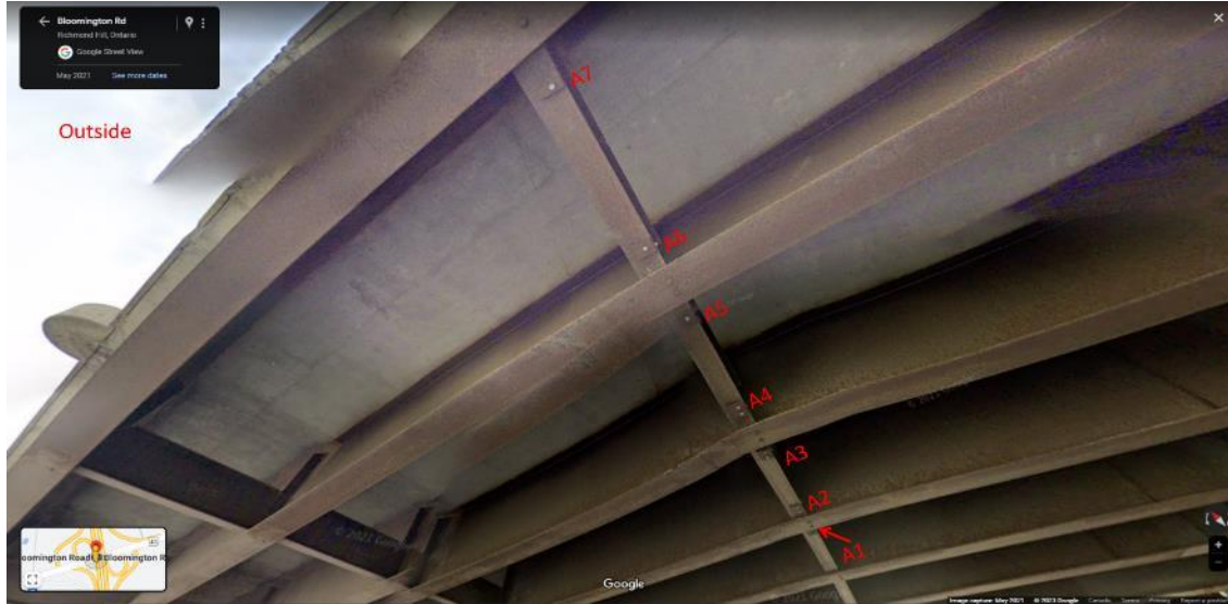
Figure 4-2. Steel plate samples installed under the Hwy 404 and Bloomington Road overpass [13].
