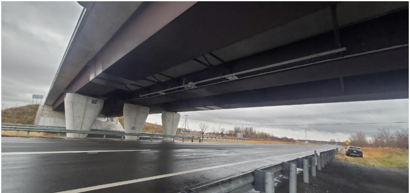
Figure 5-23. Wide-angle view of the structural monitoring system in place after the final day of installation. The image captures the sensor plates mounted across the concrete piers and the weathering steel box girders.
