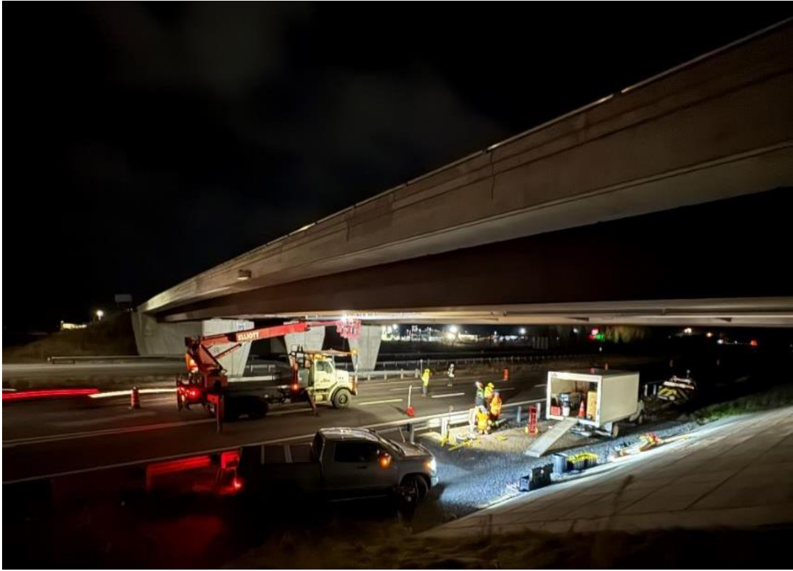
Figure 5-17. Overview of the nighttime field operations, illustrating the Highway 401 lane closure and the vehicles utilized for the transport and deployment of monitoring instrumentation.
